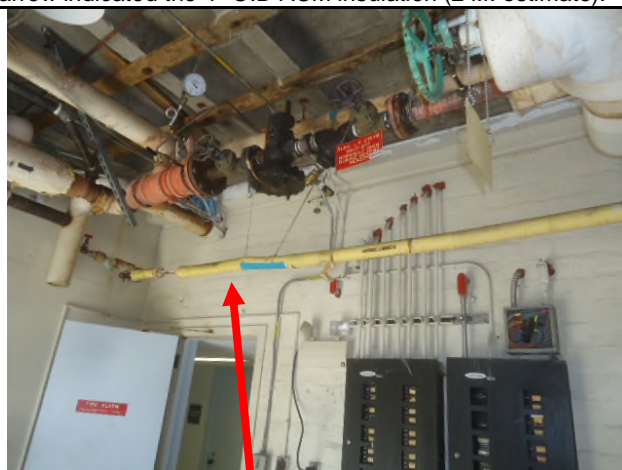
Photo 12: This is a view of the presumed 2" old pipe insulation location. The material was in bad shape and merely moving the fiberglass to expose it may have caused an asbestos clean-up. Therefore, the material is presumed ACM. (~2 l.f. estimate).
