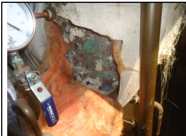
Photo 9: This is a view of the ACM insulation remnants, under the fiberglass over-lay on Tank 2.
