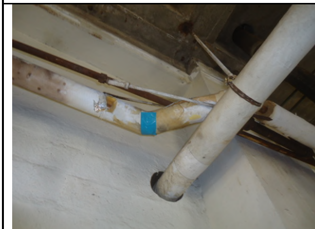
Photo 11: This is a view of the non-ACM 2" mudded elbow (just north of T-1).
