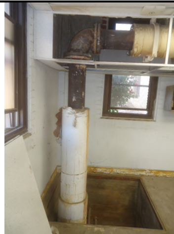
Photo 6: This is a view of the west side, where the piping again runs below grade. Outside the building, the piping must be presumed ACM and tested when exposed.
