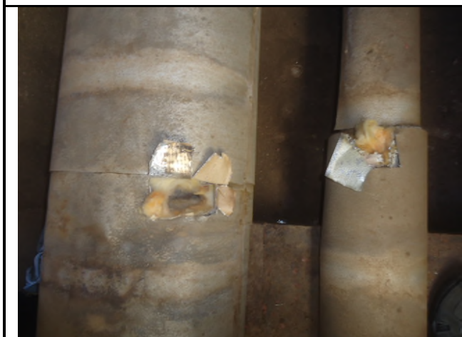
Photo 3: This is a view of the fiberglass insulation on the large diameter piping.
