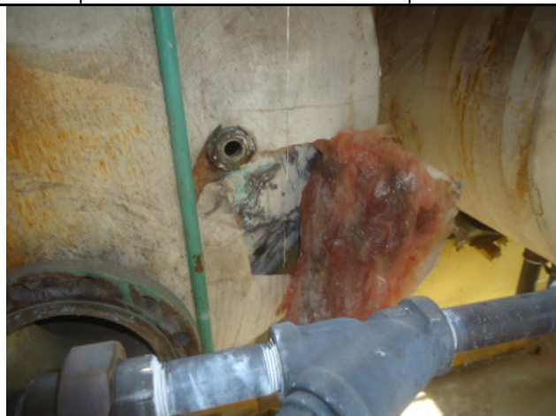
Photo 8: This is a view of the ACM insulation remnants, under the fiberglass over-lay on Tank 1. (200 s.f. per tank estimate)
