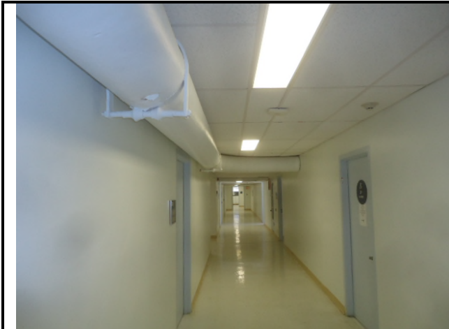
Photo 5: This is a view inside the building, of the same fiberglass insulated pipe.
