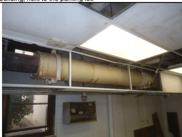
Photo 4: This is a view inside the building, of the same fiberglass insulated pipe.
