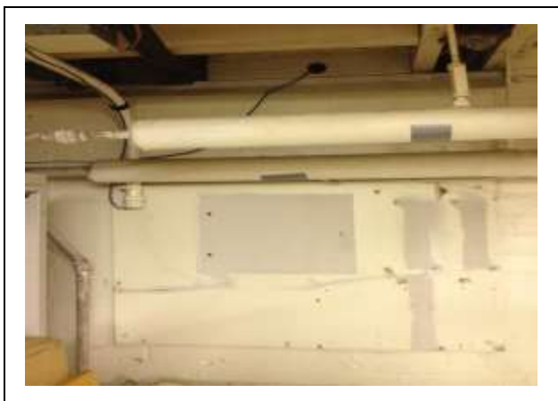
PHOTO 9 Asbestos-Containing Pipe Insulation – mag type
