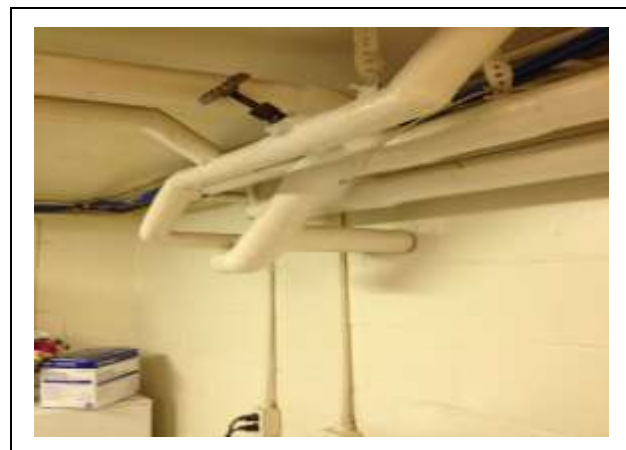
PHOTO 10 Asbestos-Containing Mechanical fitting insulation associated with air cell and mag pipe runs
