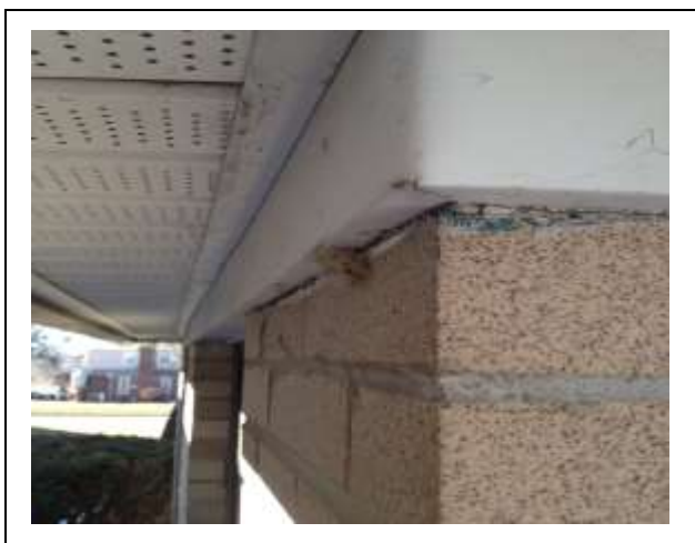
PHOTO 11 Asbestos-Containing Soffit/Roof edge sealant
