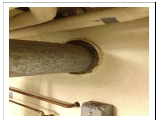
PHOTO 6 Asbestos-Containing mortar at vent pipe penetration
