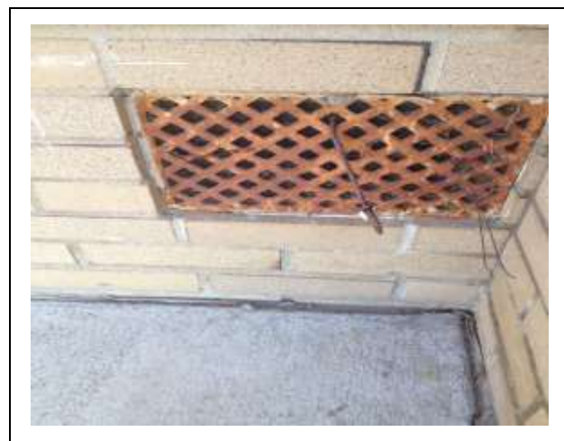
PHOTO 12 Asbestos-Containing Exterior exhaust vent sealant
