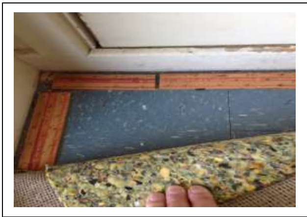
PHOTO 3 Asbestos-Containing Black mastic under 12" x 12" blue vinyl tile
