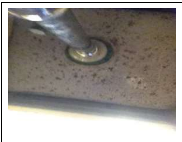
PHOTO 5 Asbestos-Containing sink undercoating
