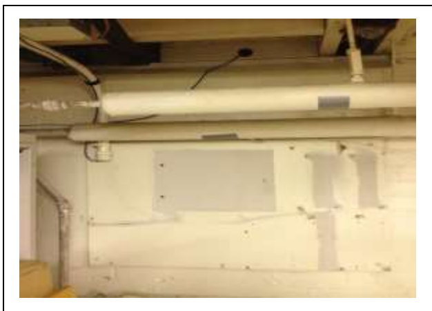
PHOTO 9 Asbestos-Containing Pipe Insulation – mag type
