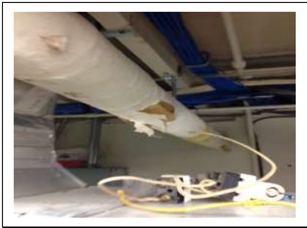
PHOTO 7 Asbestos-Containing Mechanical fitting insulation associated with fiberglass pipe runs
