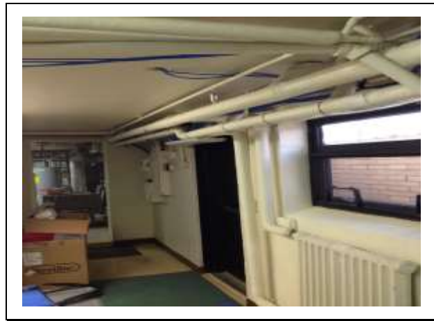
PHOTO 8 Asbestos-Containing Pipe Insulation – air cell type
