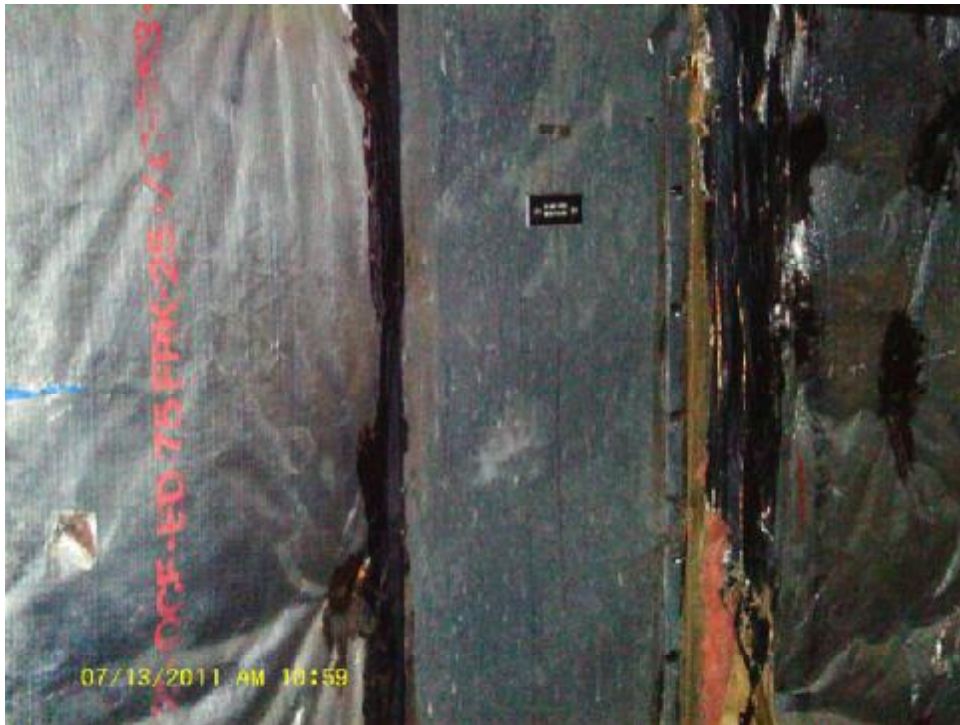
21-7 Black mastic on round duct insulation - AHU 21 3% Chrysotile in dark brown sealant
