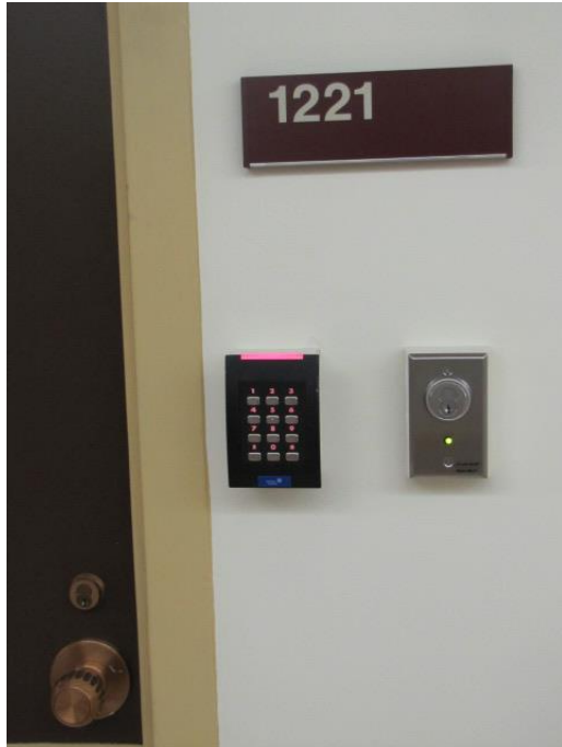
PIV Reader outside of the Data Closet Room
