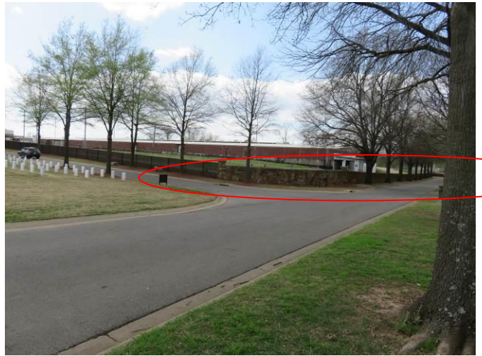
Figure 13: C1.2 (reverse) to be repaired
