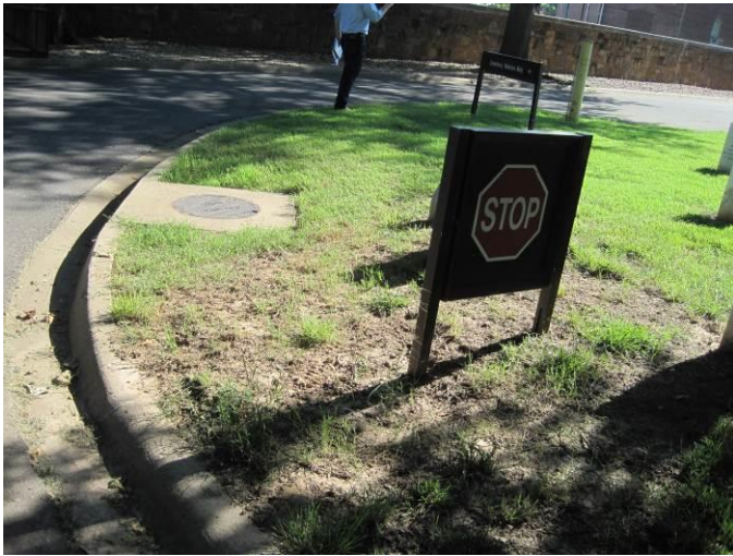
Figure 12: C1.1 to be repaired
