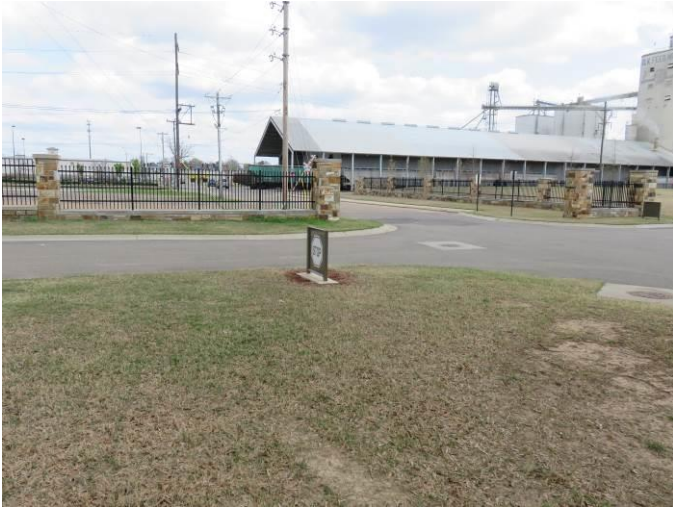
Figure 16: C1.5 to be repaired
