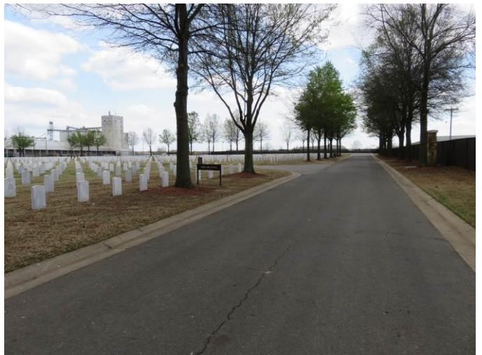
Figure 21: D2.2 to be removed and replaced
