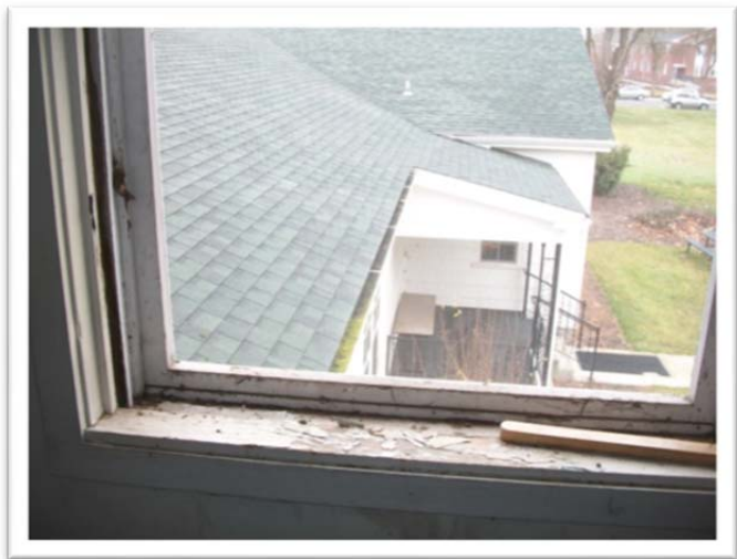
Sample 14-113A.L16, White Paint, 170,000 ppm Lead
