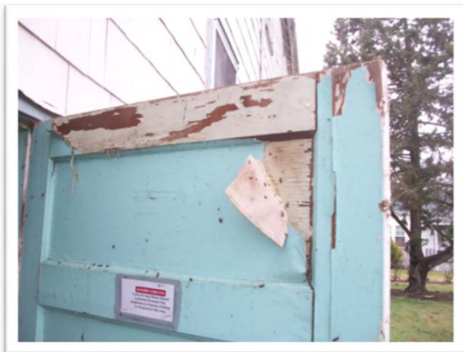
Sample 14-113A.L12, Green Paint, 6,400 ppm Lead
