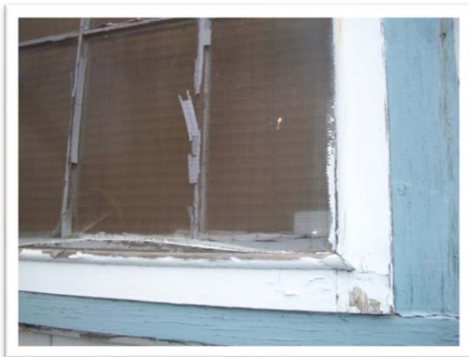
Sample 14-113A.L10, White Paint, 58,000 ppm Lead
