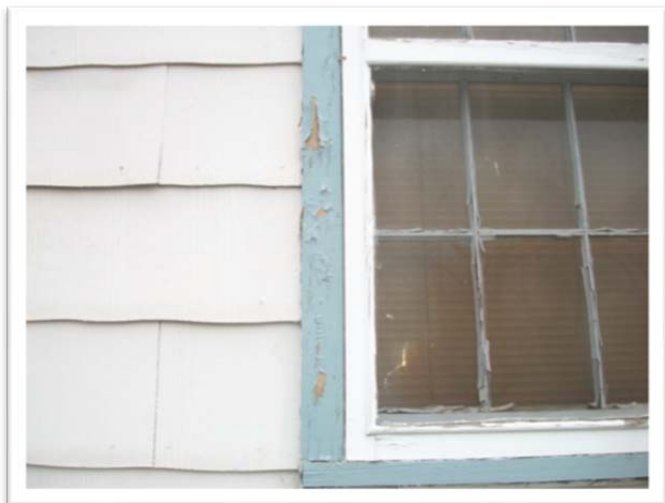
Sample 14-113A.L11, Blue Paint, 210,000 ppm Lead
