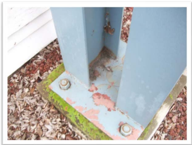
Sample 14-113A.L15, White Paint, 68 ppm Lead
