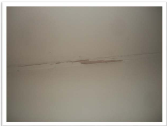
Sample 14-113A.L18, White Paint, 1,400 ppm Lead
