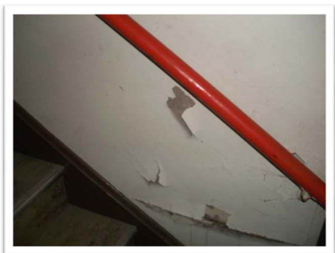
Sample 14-113A.L19, White Paint, 2,700 ppm Lead
