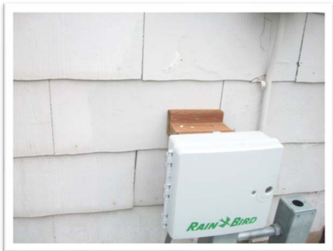
Sample 14-113A.L9, Gray Paint, 6,100 ppm Lead
