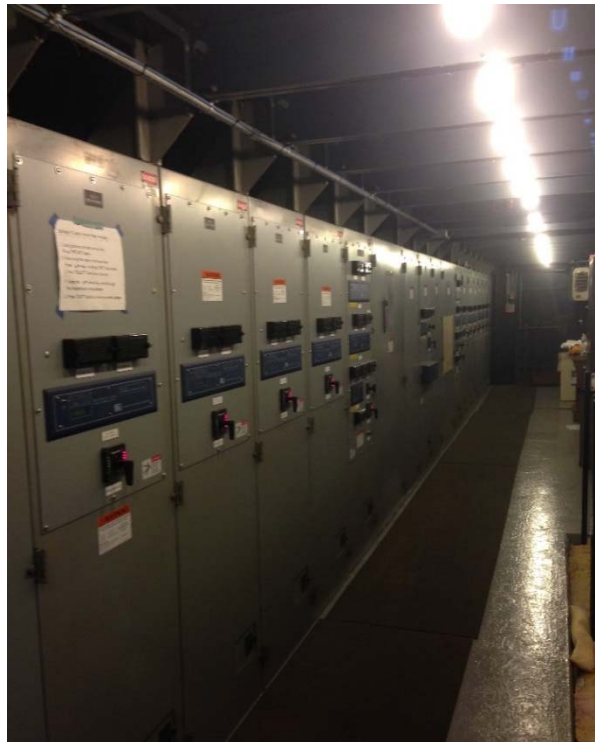
Photograph 1: Medium voltage switchgear
