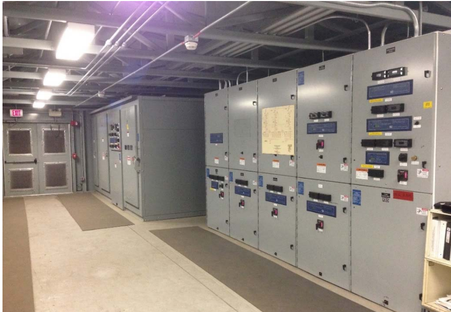
Photograph 2: Medium voltage switchgear
