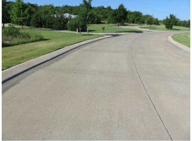
Figure 2: Lone Star Circle (typical joint layout).
