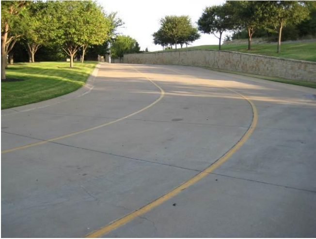
Figure 7: Shelter Drive (typical joint layout).
