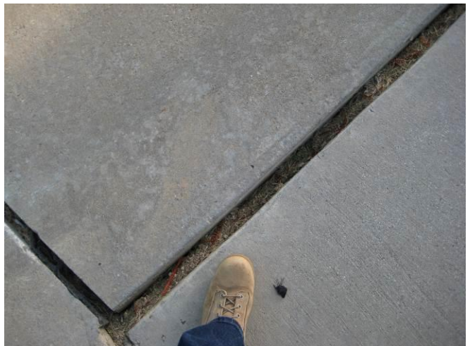
Figure 6: Example of extra wide joint (from Figure 5)
