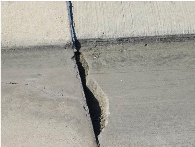
Figure 3: Example of spall near joint.
