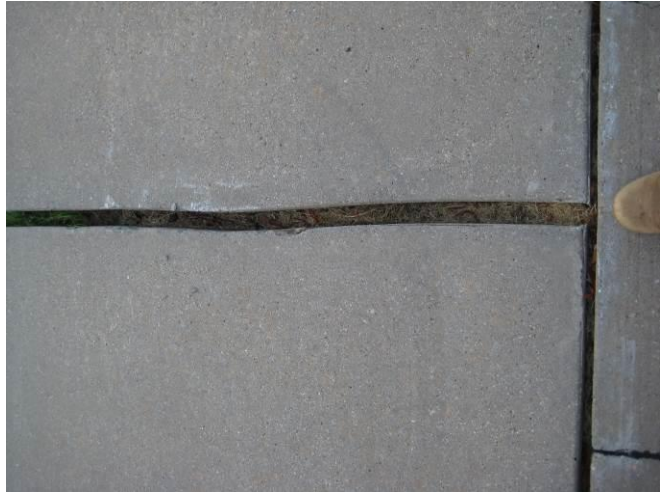
Figure 8: Example of extra wide transverse joint at Shelter Drive (boot on right for scale)
