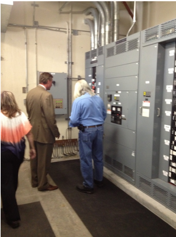
Existing MDP and EMDP in Main Electrical Room
