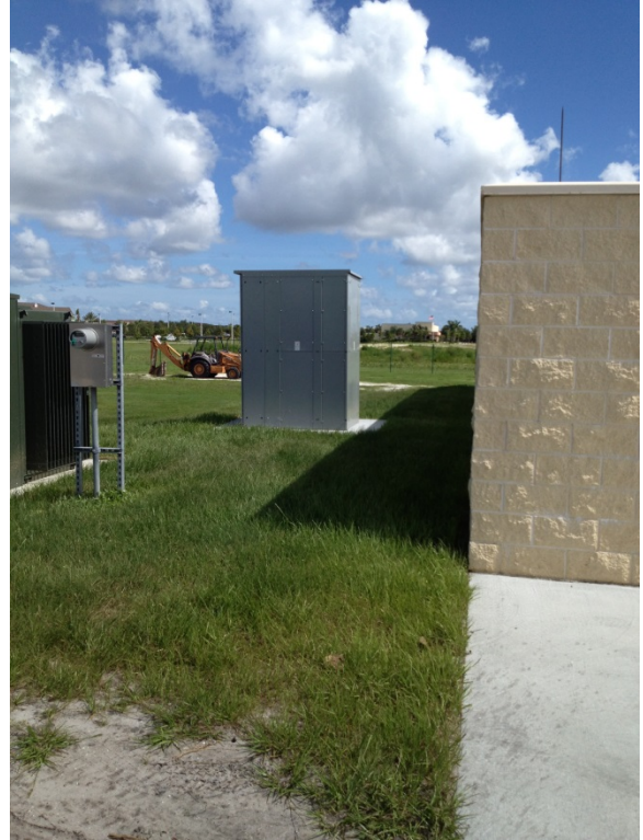
Existing utility company pad mount transformer and enclosure
