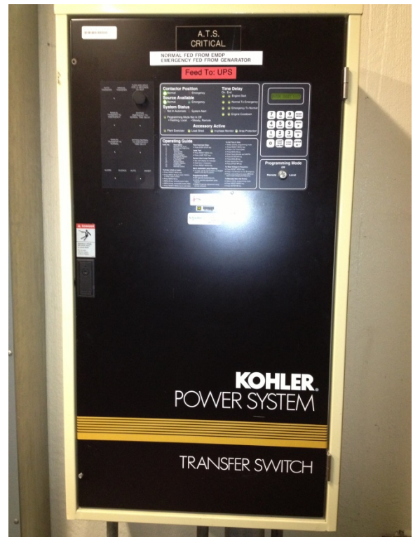
Existing ATS Critical in Main Electrical Room
