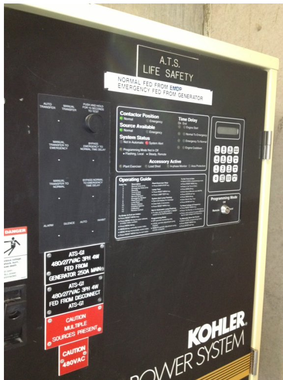
Existing ATS Life Safety name plate data
