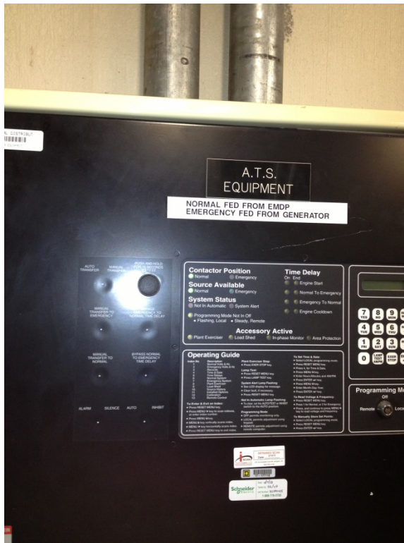
Existing ATS Equipment in Main Elect. Rm.
