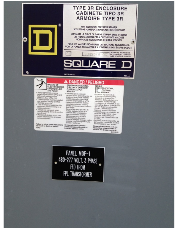
Existing MDP-1 nameplate in Chiller Plant
