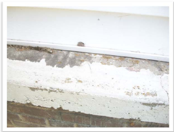
Sample 15-090A.L7, Cement Sill, 110 ppm Lead
