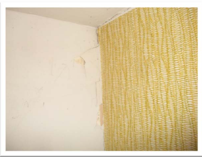
Sample 15-090A.L4, Wall Paint, 1,600 ppm Lead
