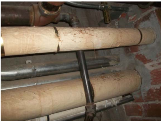
15-090A.19, Pipe Insulation, 20% Asbestos (Lowest Pipe)
