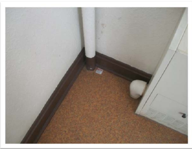
15-090A.40, Red Vinyl Floor, 30% Asbestos
