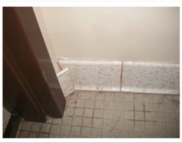
15-090A.33, 1" Ceramic Tile, Non-ACM 15-090A.34, Ceramic Base, Non-ACM
