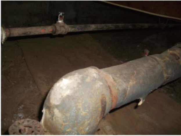
15-090A.13, Pipe Insulation, 50% Asbestos
