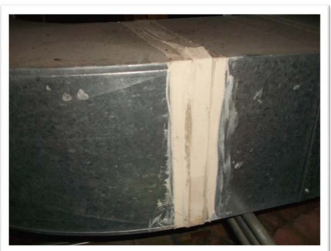
15-090A.12, White Duct Tape, Non-ACM
