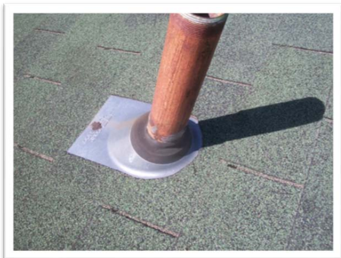
15-090A.3, Roof Sealant, 5% Asbestos
