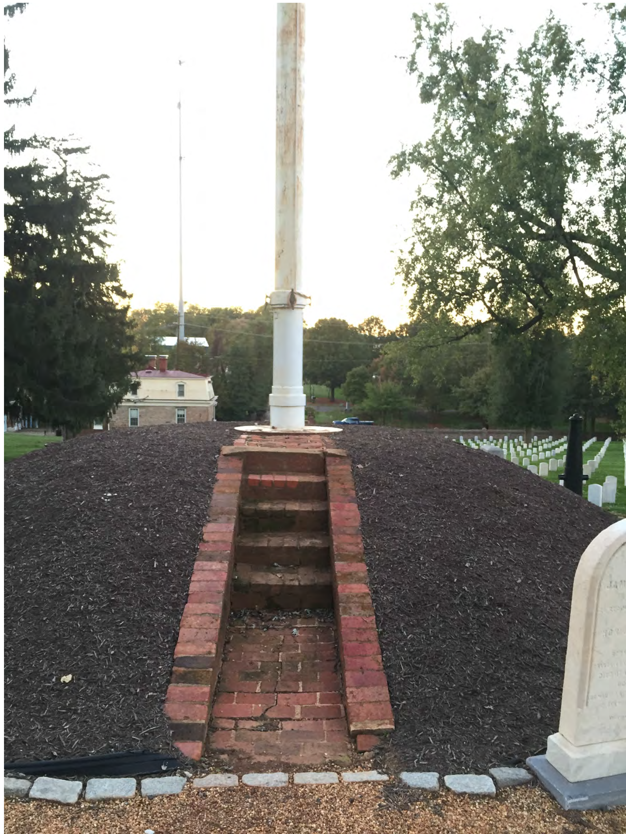
Detail 3: Carefully remove entire existing walled brick walkway and stairway and reinstall existing bricks with new type S mortar. Excavate and compact a new 6" subbase of aggregate under all brick rework. Remove existing mulch from, stone paver edging, and gravel. Note this area is a burial area and a headstone can be seen at the right lower portion of this picture. Protect burial markers in place during all work. The mulched area is also to be treated as a burial area. Prepare subgrade and install 4" of new topsoil and new sod in the formerly mulched and graveled area.
