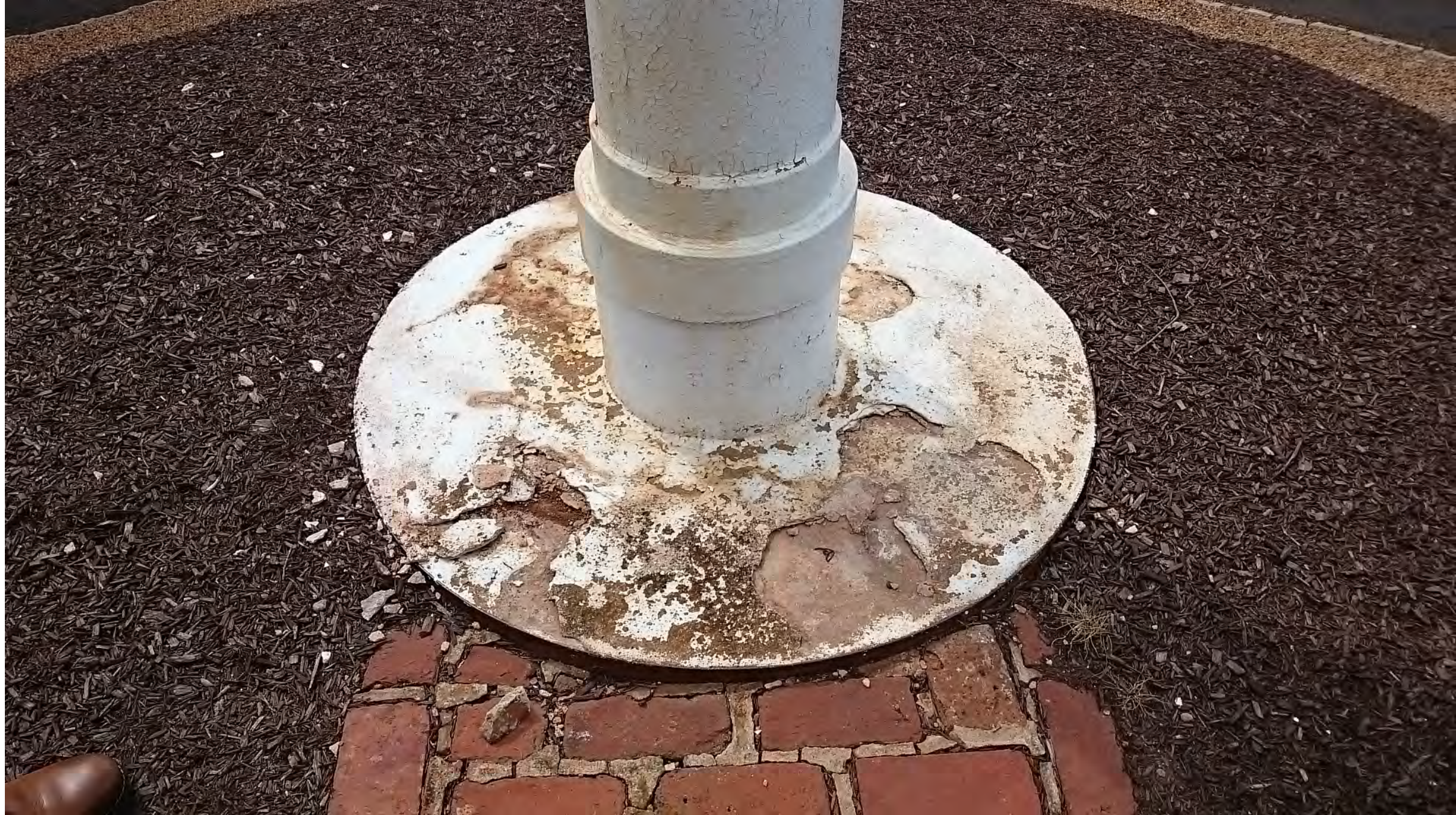
Detail 4: Demolish existing mortar at flagpole base and install new mortar. Slope new mortar away from flagpole towards mulch bed. Paint new mortar to match newly painted flagpole.
