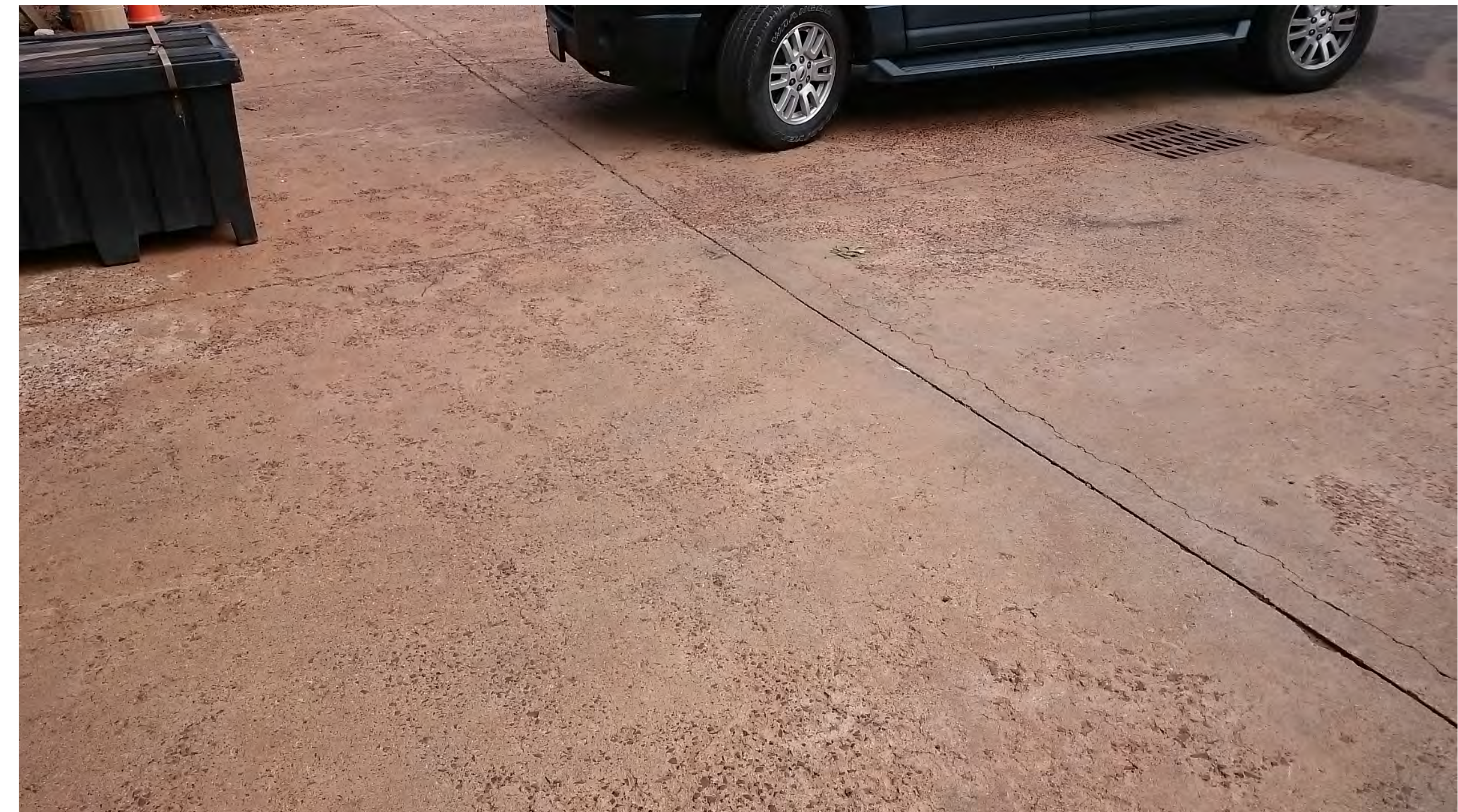
Detail 2: Picture showing condition of concrete slab to be replaced at maintenance complex.
