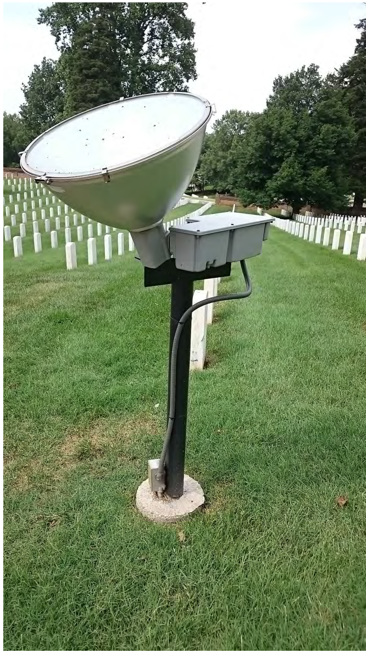
Detail 1: Demolish existing floodlight fixture and replace with new LED fixture. Four (4) locations. Reuse existing foundation and steel base and cabling/conduit. Install new photocell to control all four (4) new LED fixtures such that they only illuminate during night.
