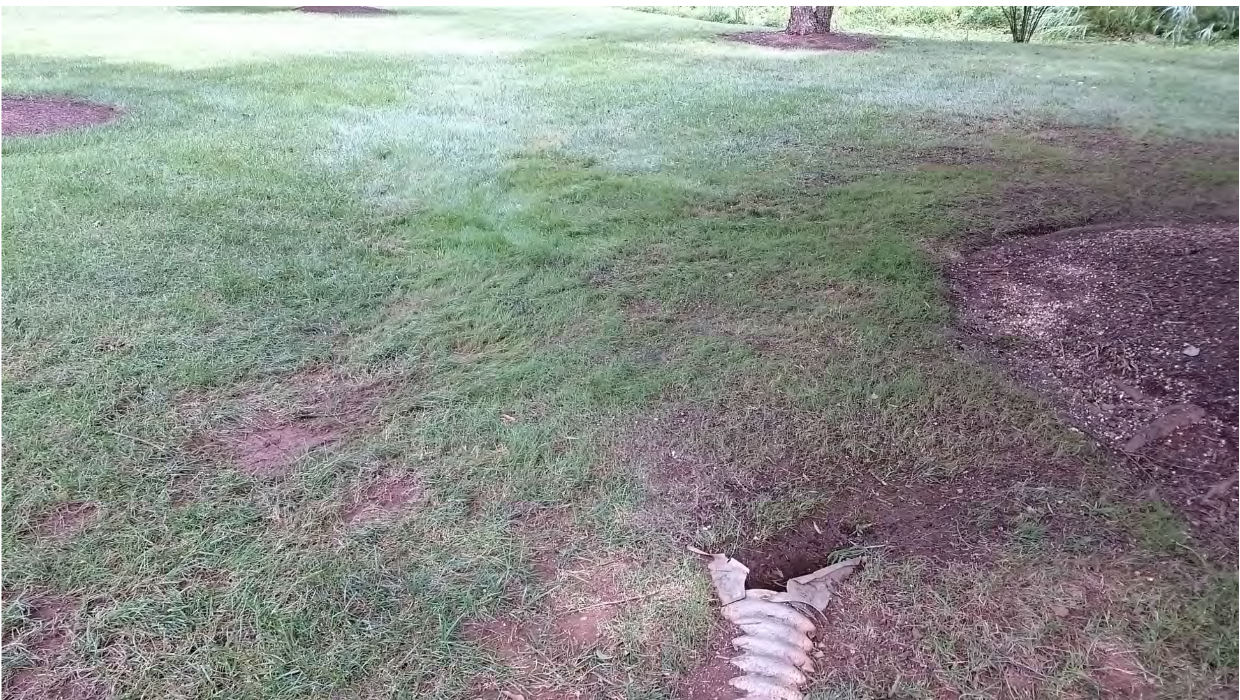
Detail 4: This picture shows the existing underdrain outlet which is just off the east side of the road that the drain runs under. The new underdrain route will extend past this outlet and to the river seen at the very back of this picture.
