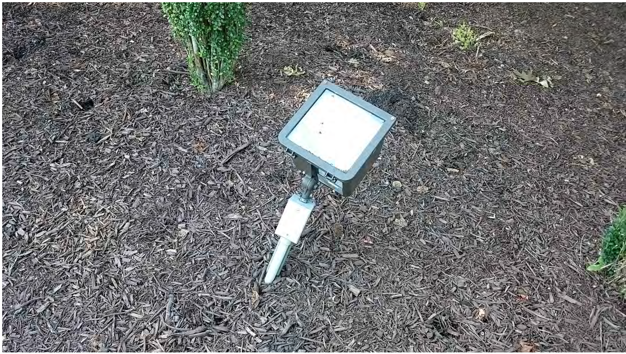
Detail 2: Demolish existing floodlight fixture and replace with new LED fixture. Three (3) locations. Install new 2'x2'x6" thick concrete foundation for the new fixture. Foundation shall be 2" above finished grade. Install new photocell to control all three (3) new LED fixtures such that they only illuminate during night.
