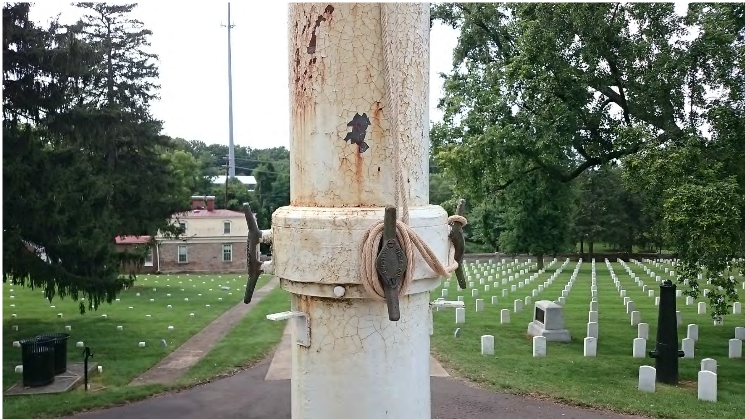
Detail 5: This picture shows the general condition of the existing flagpole and paint. Strip paint, prep surface, and install new paint per specifications.
