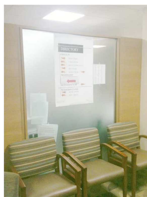
2 PARTIAL HEIGHT PARTITION - SALVAGE AND REUSE SCALE: NTS
