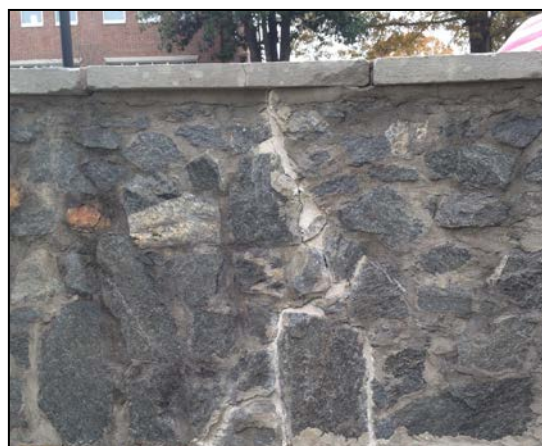
Figure 2. Unacceptable stone repair.
