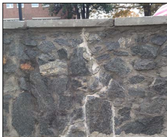
Figure 2. Unacceptable stone repair.
