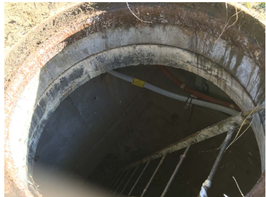
FIG #1: 12KV CIRCUIT A-1 FROM SUBSTATION INSIDE MANHOLE "MH-2".
