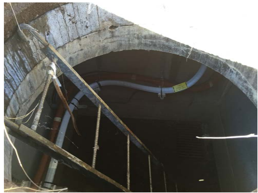
FIG #2: 12KV CIRCUIT A-1 TO SWITCHBOARD 138A INSIDE MANHOLE "MH-2".
