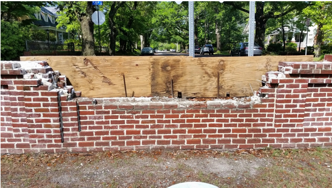
Figure 2 above: View of damaged brick wall from inside the cemetery.
