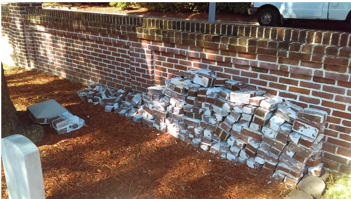
Figure 4 above: This picture shows existing bricks and the damaged column top loose on the ground, to be utilized for the repairs. It also shows the existing wall and a bit of an existing column in the upper left of the picture, to which repairs are to match.
