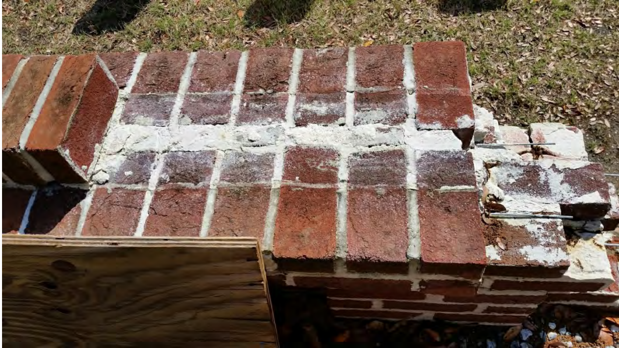
Figure 5 above: This picture shows the general construction of the brick wall including reinforcement, width and arrangement of bricks.
