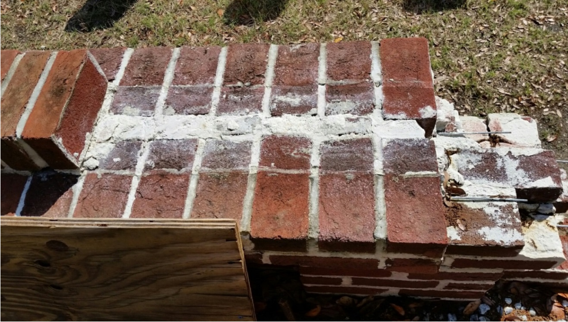
Figure 5 above: This picture shows the general construction of the brick wall including reinforcement, width and arrangement of bricks.
