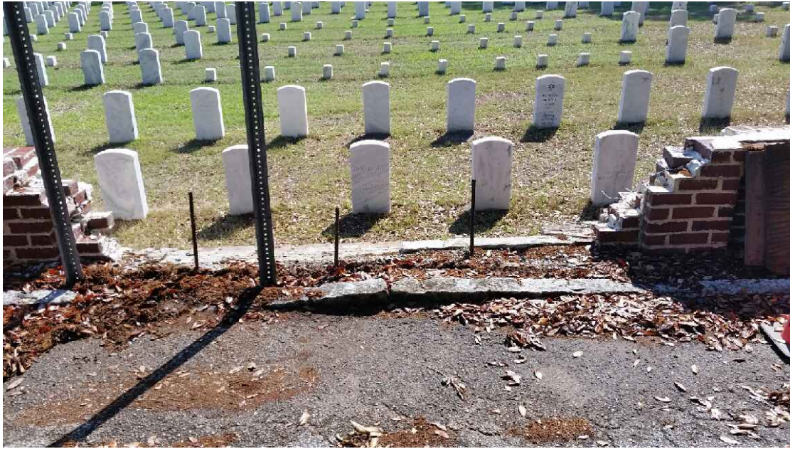
Figure 1 above: View of damaged brick wall from outside the cemetery. Note the asphalt road and curb are at a higher elevation than the cemetery burial area on the other side of the wall. Utilize the existing vertical reinforcing bars in the repair work for structural strength. Splice existing reinforcing bars with new new reinforcing bars of the same size up to the full height of the replaced wall following ACI 301 standards and use ASTM A 615/A 615M, Grade 60, deformed reinforcing steel.
