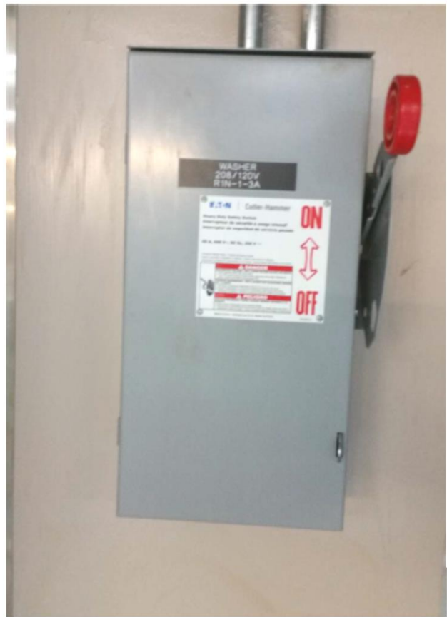
Disconnects (208/120V) for each machine on non-sterile side
