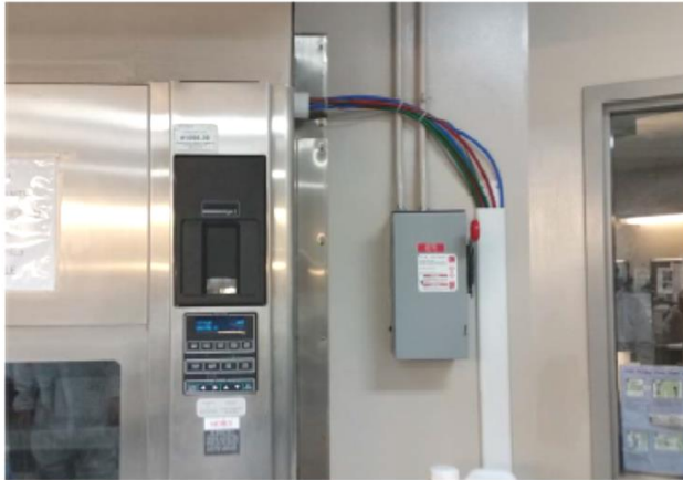
Non-sterile side of machines, and locations of disconnects
