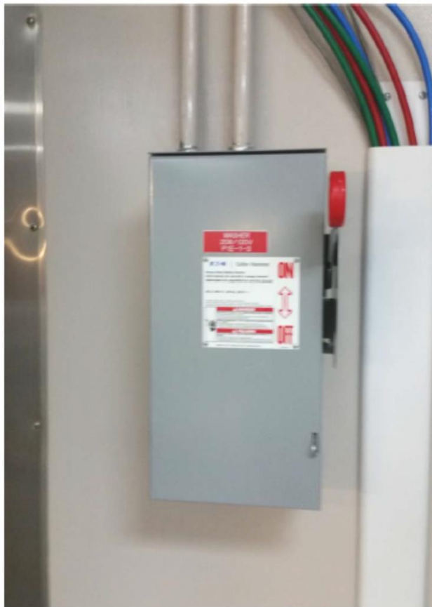
Disconnects (208/120V) for each machine on non-sterile side
