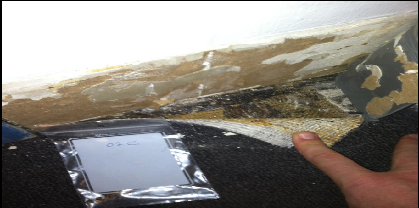
Building 1 - Conference Room Carpeting and Mastic
