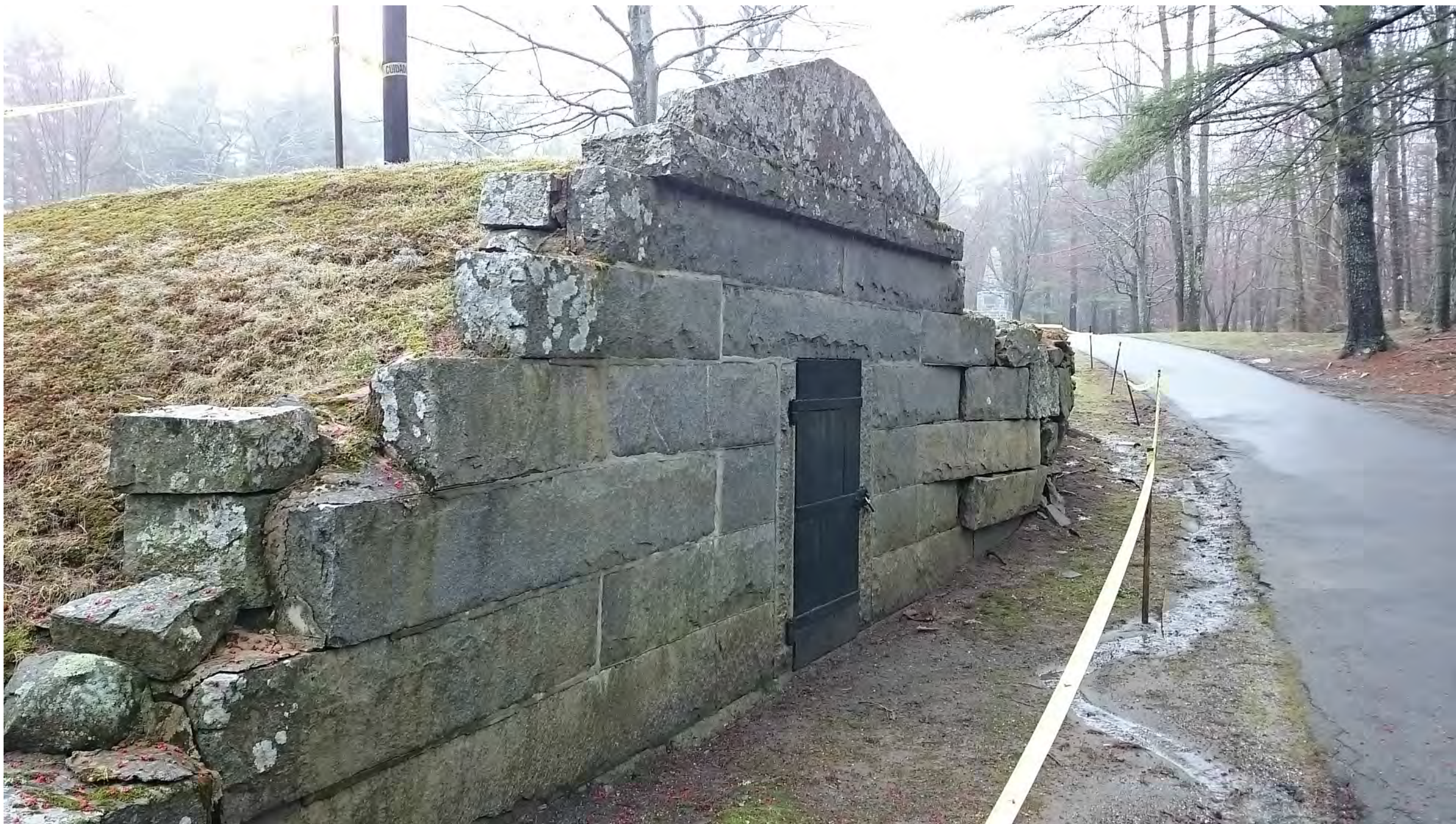
Detail 1: Remove stones and mortar. Protect and support existing earth, masonry mausoleum, door. Install existing stones with new mortar to match existing in appearance. Demolish foundation and earth as necessary. Design and build a reinforced concrete foundation to be hidden from view below grade.
