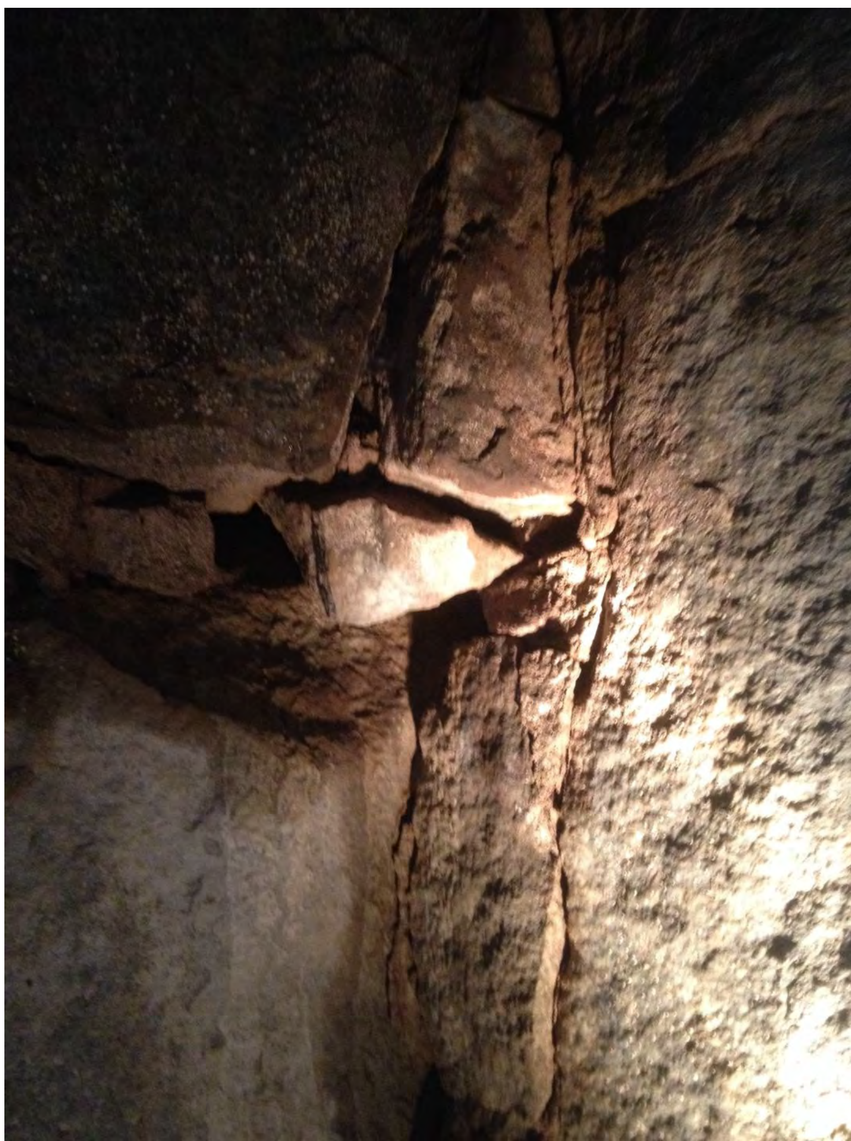
Detail 5: Picture showing interior stone wall of the mausoleum and a specific failure. Remove existing stones, and save for reuse. Remove existing mortar. Install existing stones back into wall with new type S mortar.
