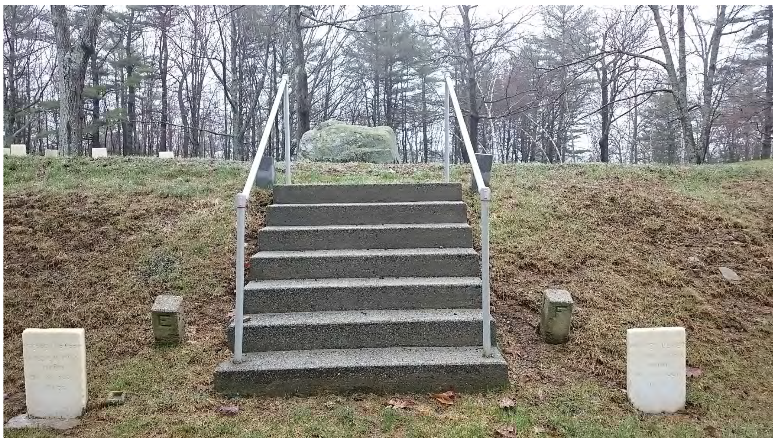
Detail 6: Epoxy the loose railing post into the stair slab. There is one (1) loose railing post.
