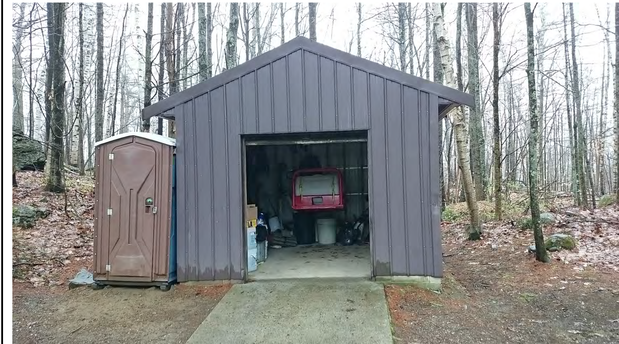
Detail 1: Picture shows one of the existing maintenance sheds which are to be demolished and a new prefabricated metal building installed. Coordinate with COR for removal of equipment from inside of the existing shed. New shed shall match existing in size so as to reuse the existing concrete slab foundation. New entry garage door shall match the width of the existing concrete slab entry drive.
