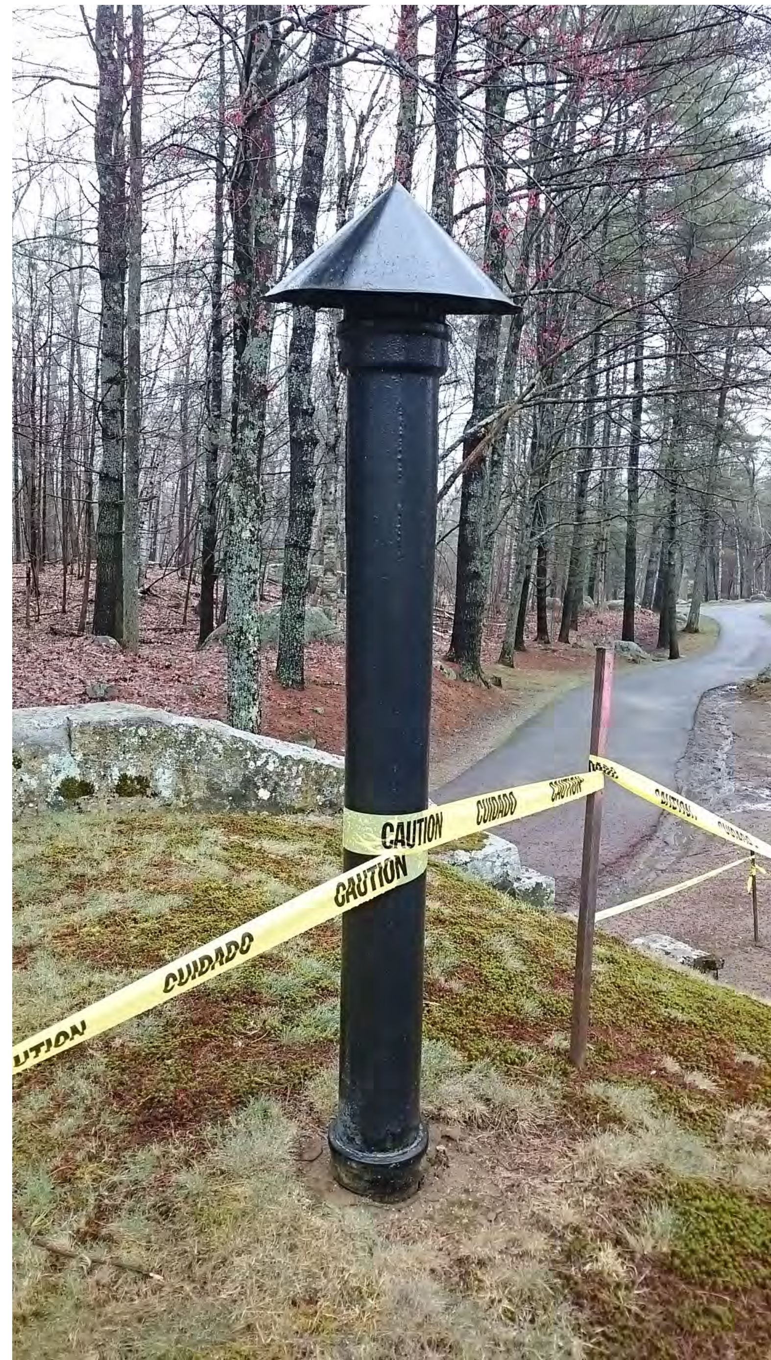
Detail 7: This picture shows the existing vent out of the mausoleum which shall be protected in place during construction. Also shown is the earth and grass cover over the existing ceiling and roof of the mausoleum.
