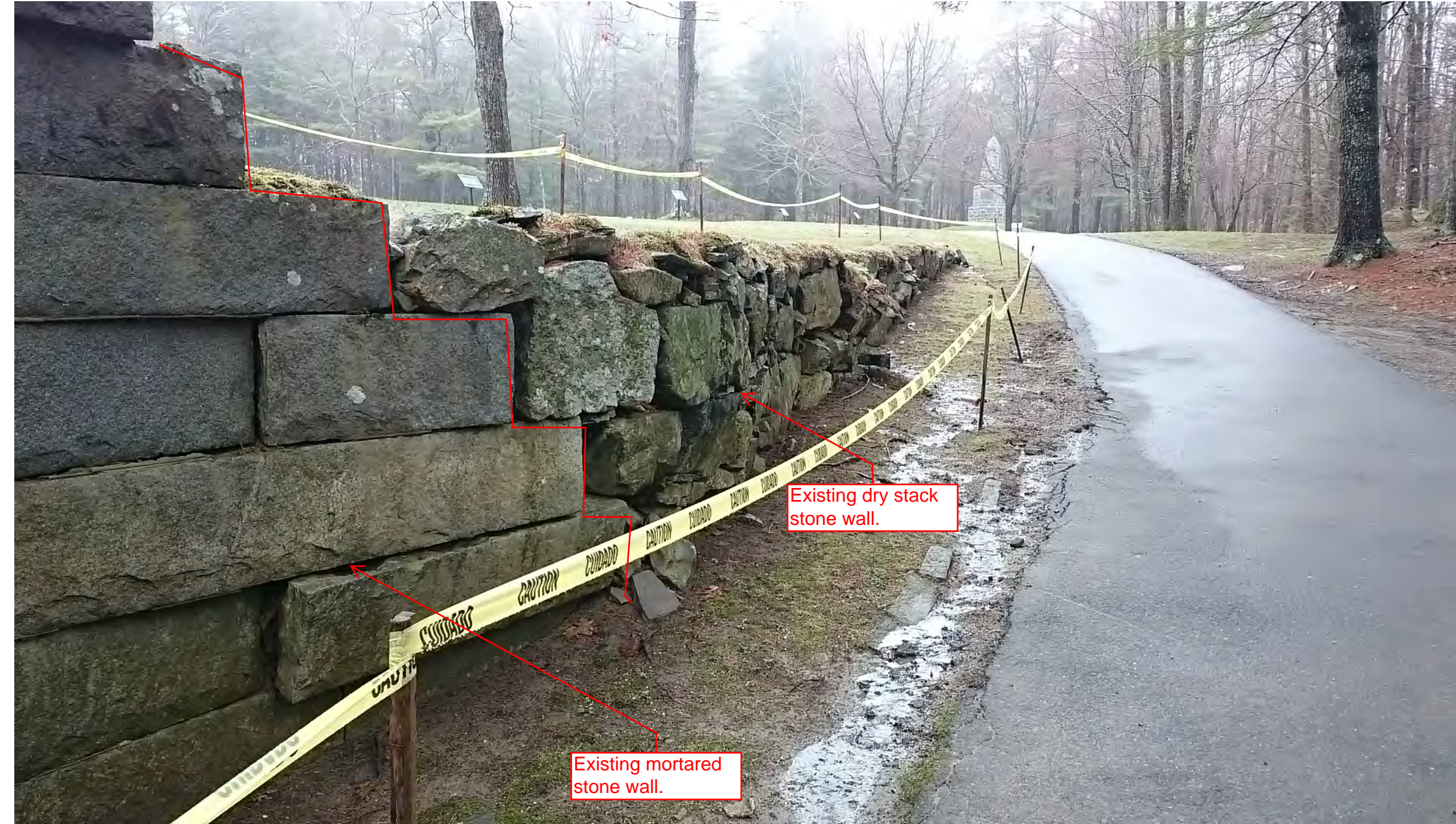
Detail 3: This picture delineates the wall repairs into two specific work scopes. The first is the area left of the red stepped line denoted as "Existing mortared stone wall." The second is the area right of the red stepped line denoted as "Existing dry stack stone wall."
