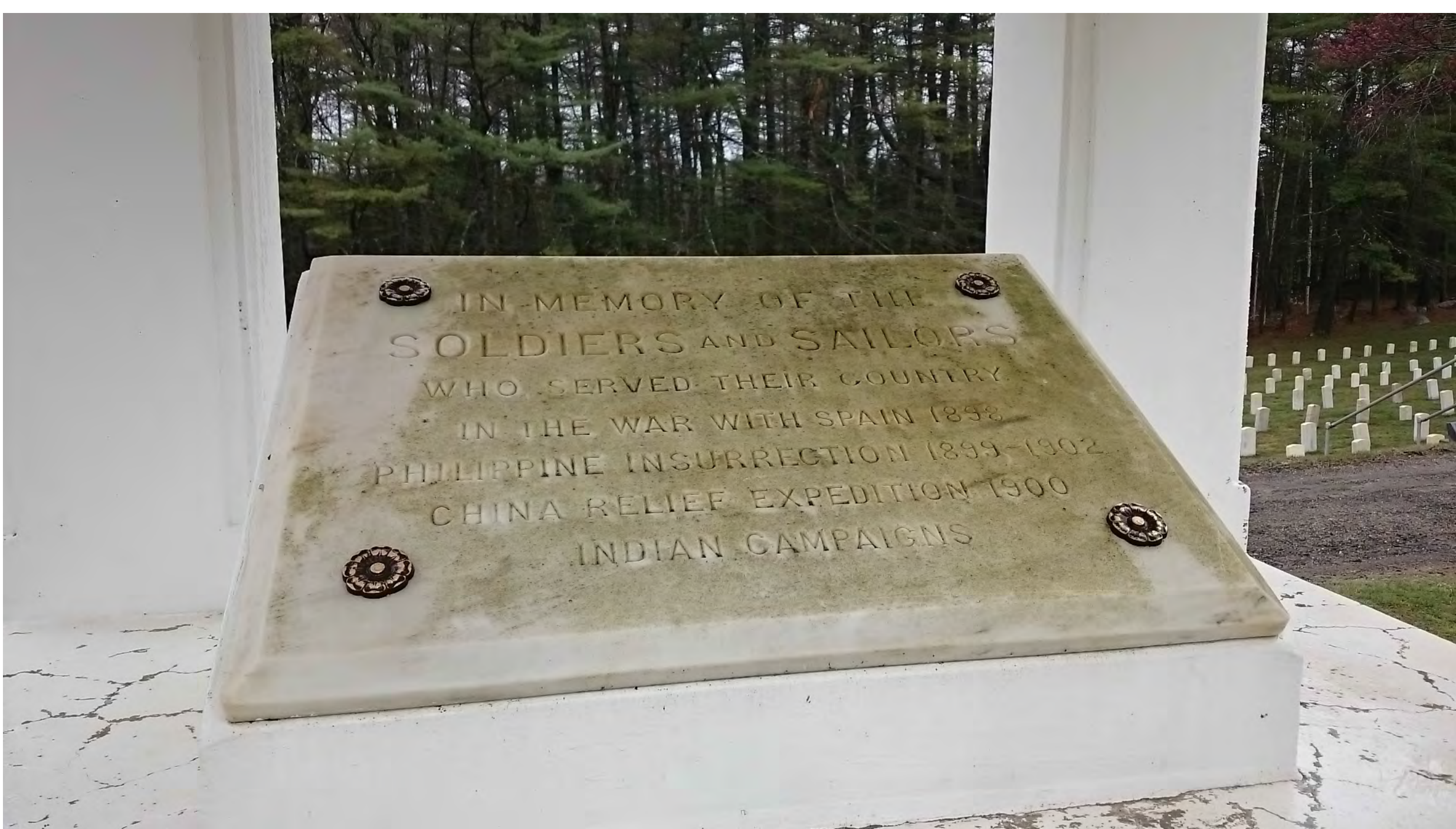
Detail 5: Clean the pictured monument tablet, which is a part of the monument shown in detail 4. Repaint. Reference specifications for more information.
