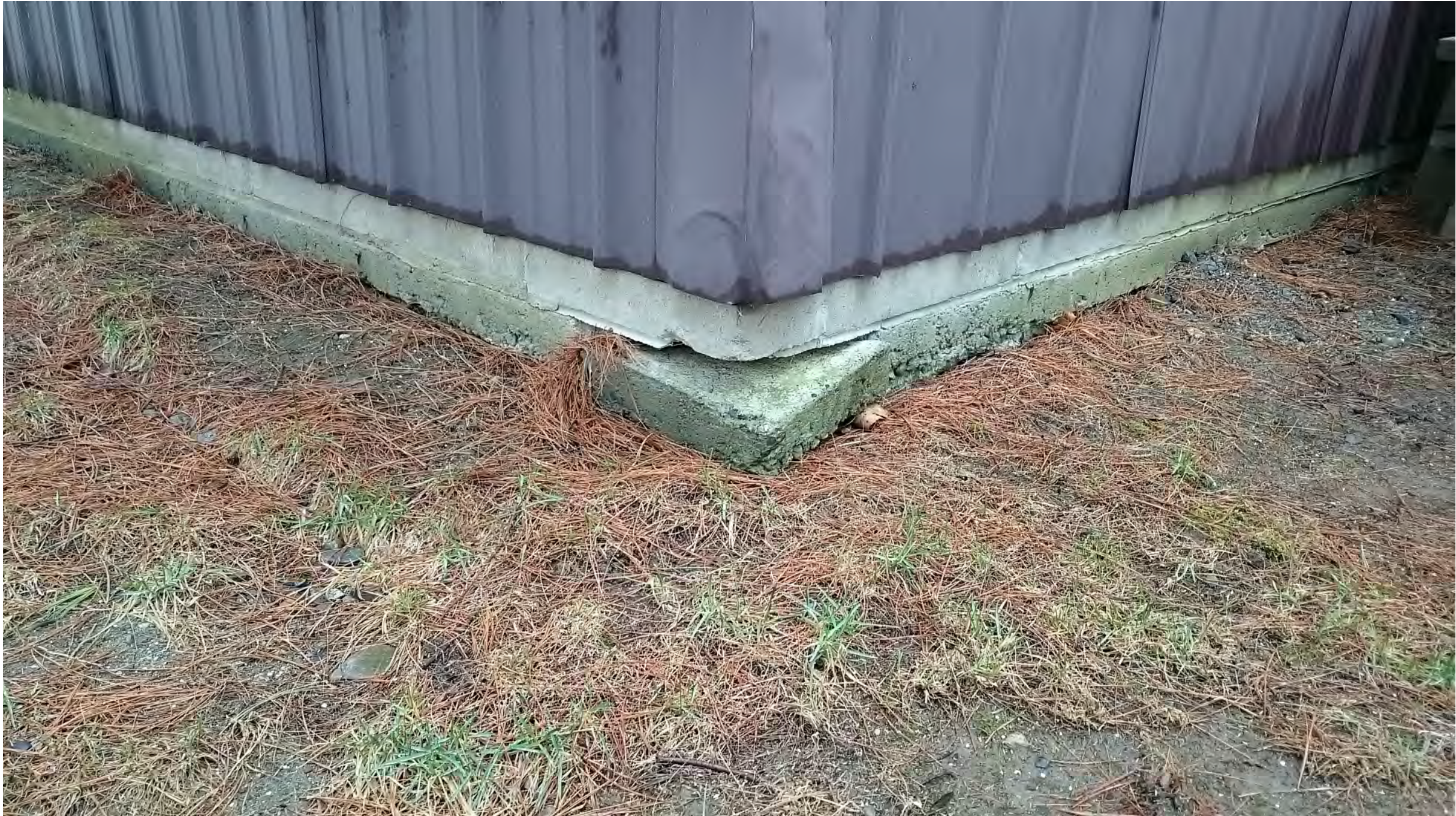
Detail 3: Remove failed corner of slab foundation to the extent necessary to patch with new concrete. Epoxy dowel #4 rebar at a minimum of every 8" into existing slab and pour new concrete. Install 8" of crushed compacted stone under this repaired section.
