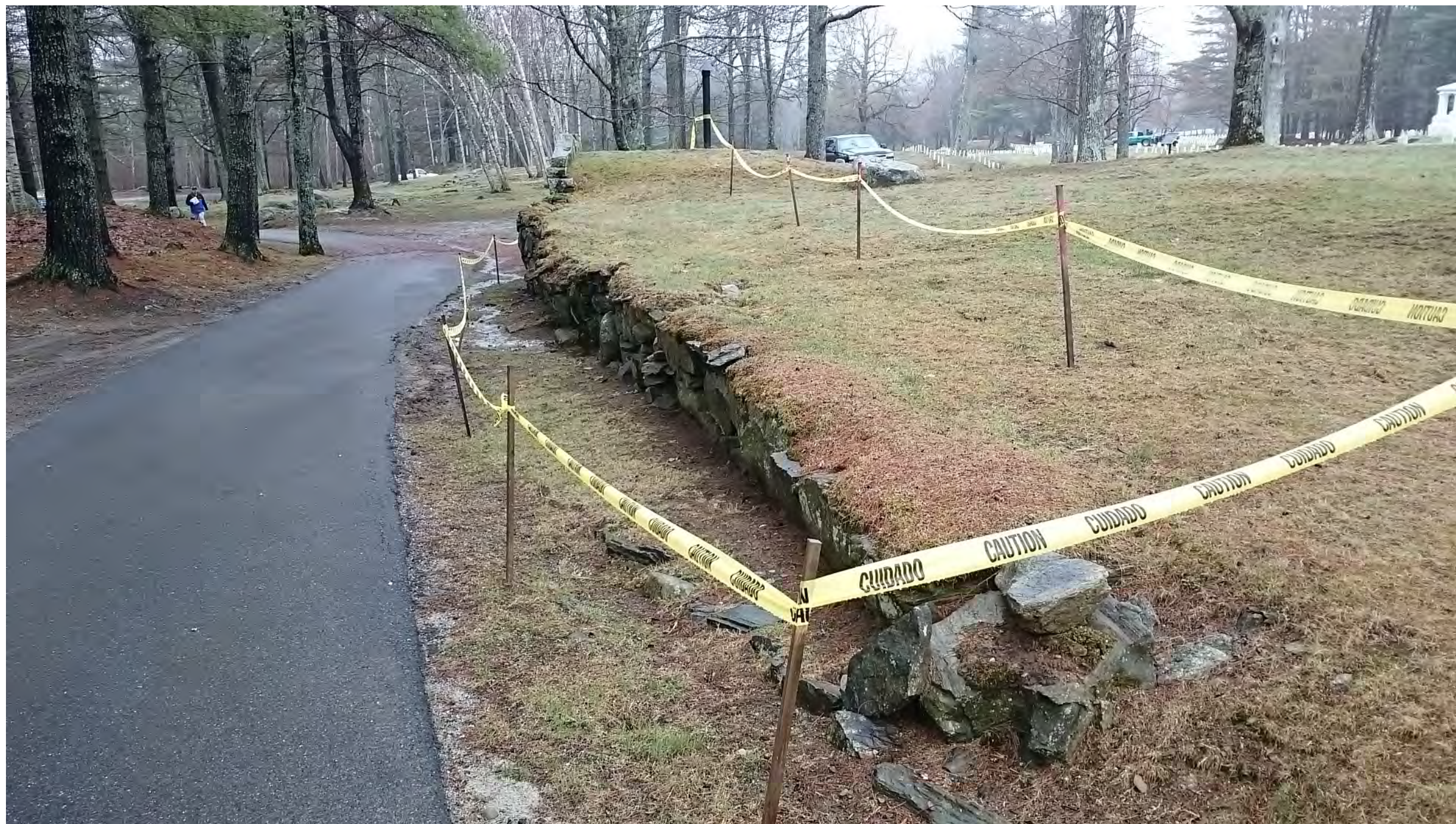
Detail 2: This picture shows the failing dry stack stone wall. Remove and protect stones. Protect and support existing earth. Install existing stones with new mortar hidden from view to match existing in appearance. Demolish foundation and earth as necessary. Design and build a reinforced concrete foundation to be hidden from view below grade.
