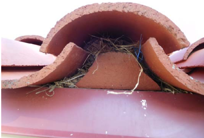
Figure 20: Example of eave closure with debris
