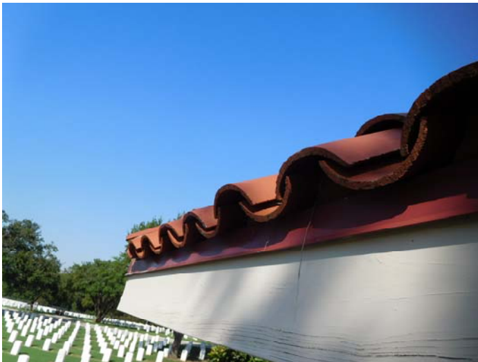
Figure 13: Example of trim board, flashing and eave
