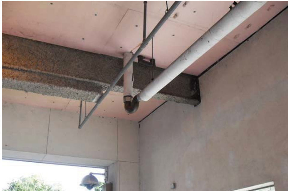
Figure 2 – Pipe insulation to be replaced.
