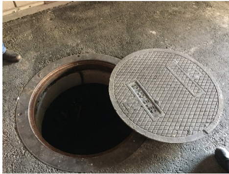
Photo #4: Medium-Voltage Vault Manhole Cover (Vault is dry inside)
