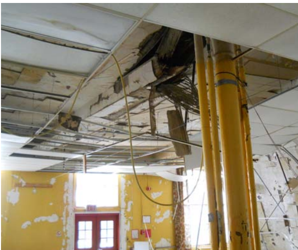
PARTIALLY COLLAPSED FIRST FLOOR TRUSS FROM NORTHEAST
