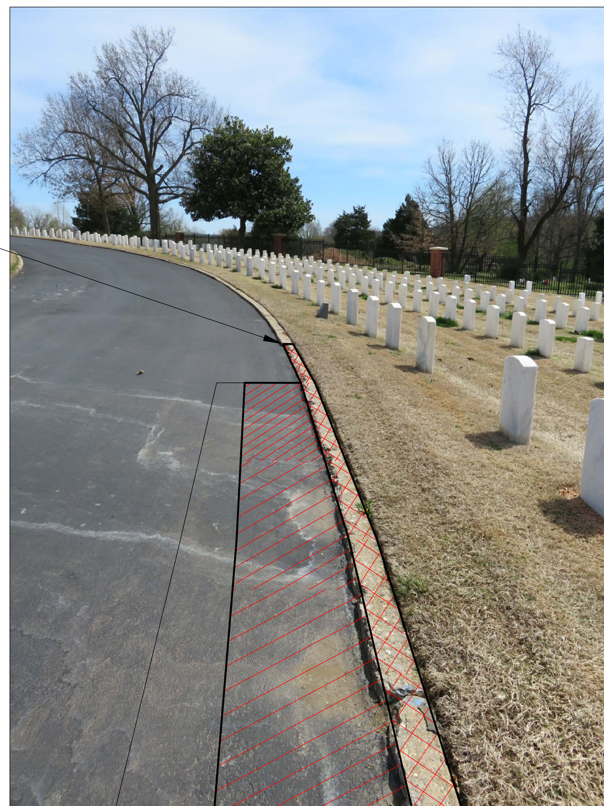
REPLACE CURB TO NEXT JOINT
