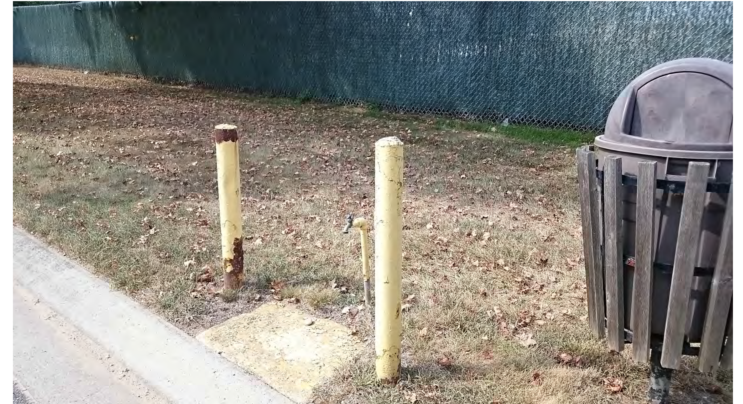
Detail 2: Picture showing the existing installations and conditions. Demolish all bollards, slabs, spigots, piping, trash cans, foundations, and structural supports either entirely or back to the specific point noted on other details and work descriptions.
