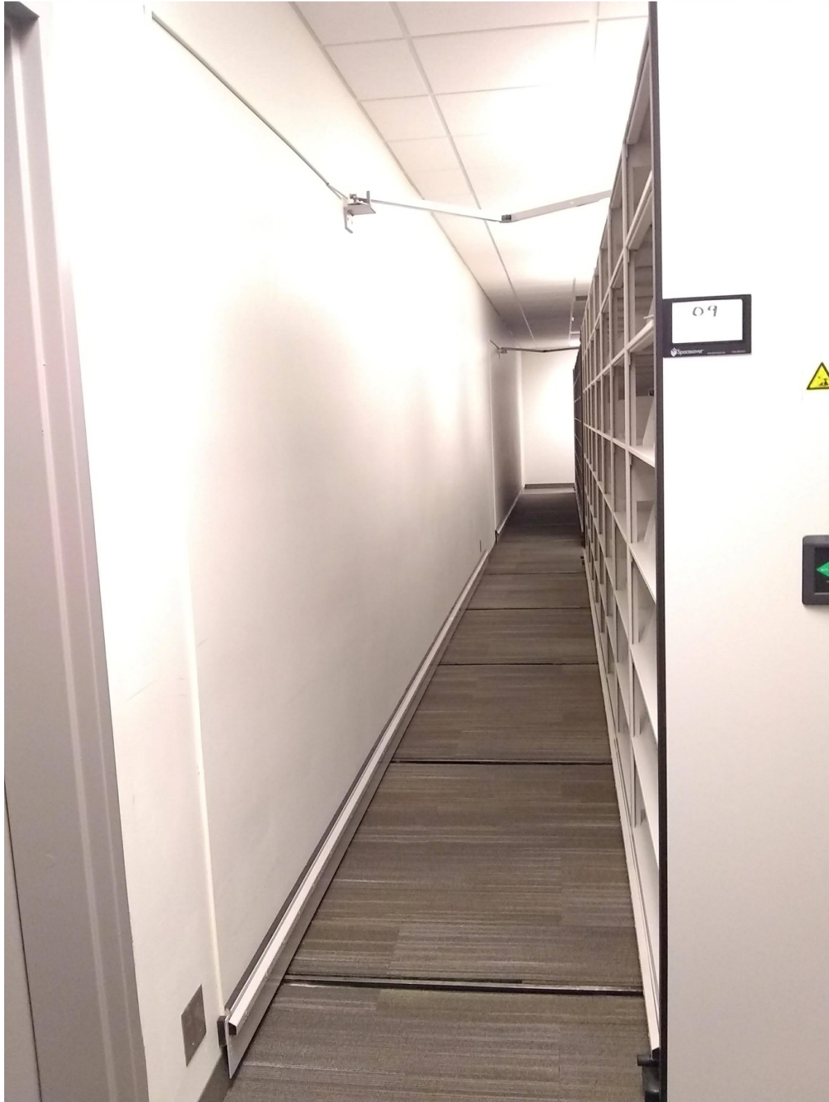
FIGURE 6: HDMS WALL HARDWARE AND FLOOR TRACKS (BASEMENT)
