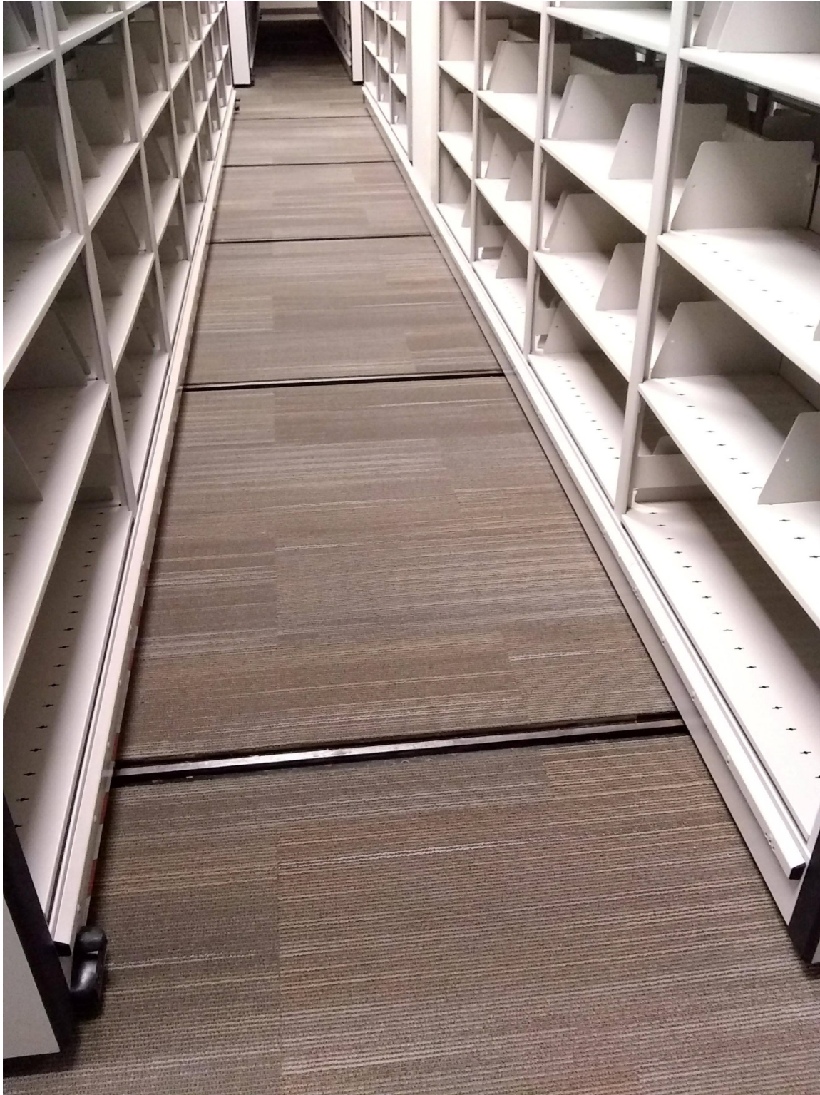
FIGURE 9: CLOSEUP OF FLOOR TRACKS (BASEMENT)
