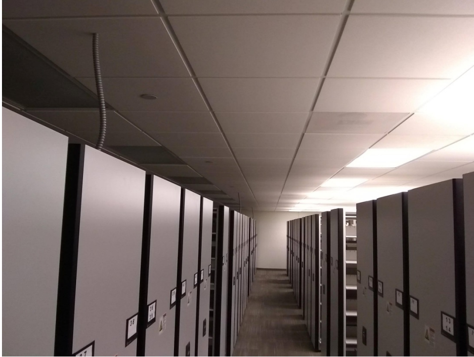
FIGURE 7: HDMS SHOWING CEILING ELECTRICAL CONNECTION (BASEMENT)
