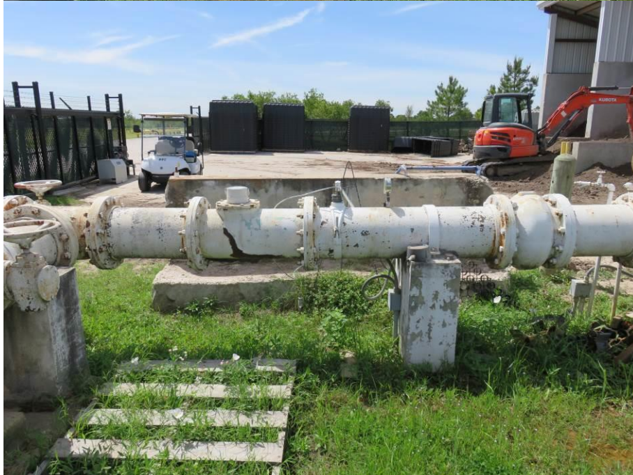
Figure 1: Western limits of work (protect circled pump motor from damage)
