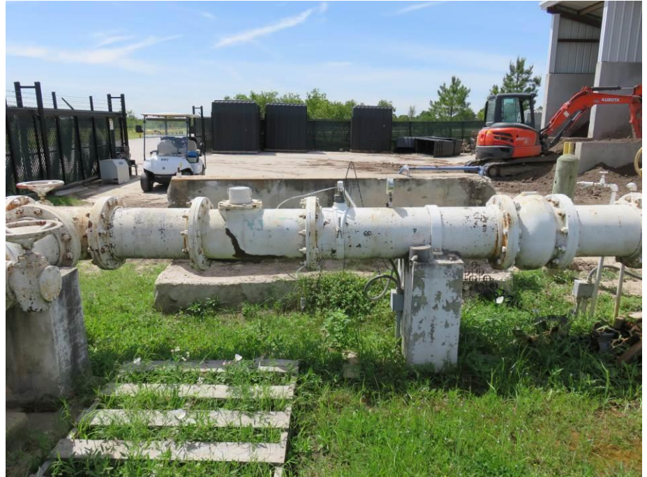
Figure 2: Distribution piping (protect water meter, center)
