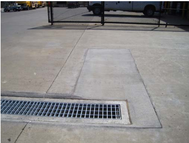
Figure 3: Existing trench drain to connect (at tie-in point)
