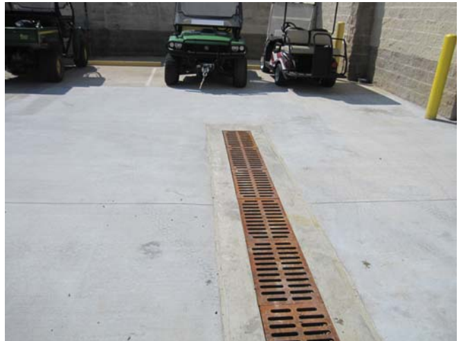
Figure 4: Existing trench drain to the North (model and basis of this design)
