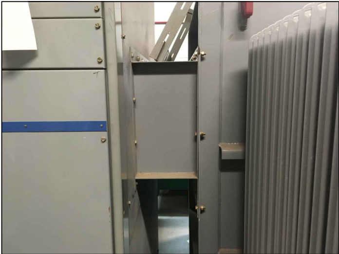
EXISTING SUBSTATION TRANSFORMER LOW VOLTAGE BUSHINGS TRANSITION PIECE
