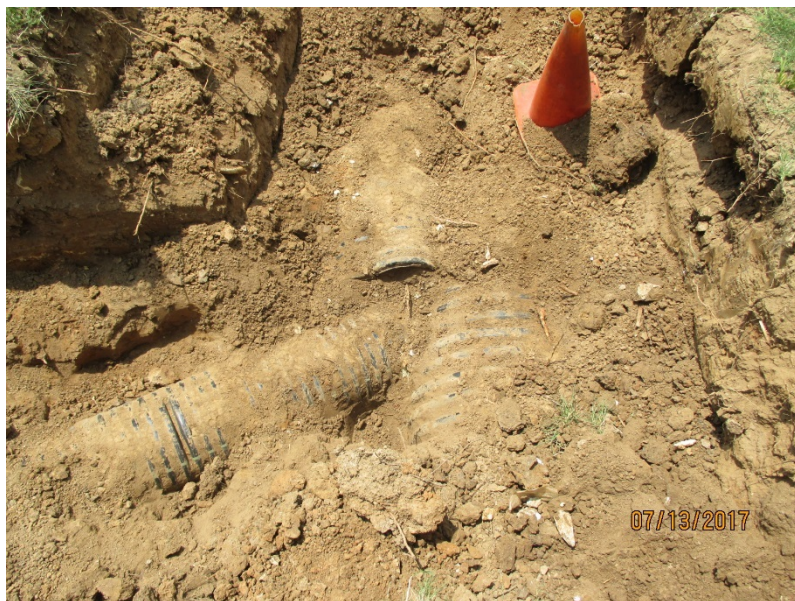
Existing Connection Point of 12" ADS Pipe to 24" ADS Pipe
