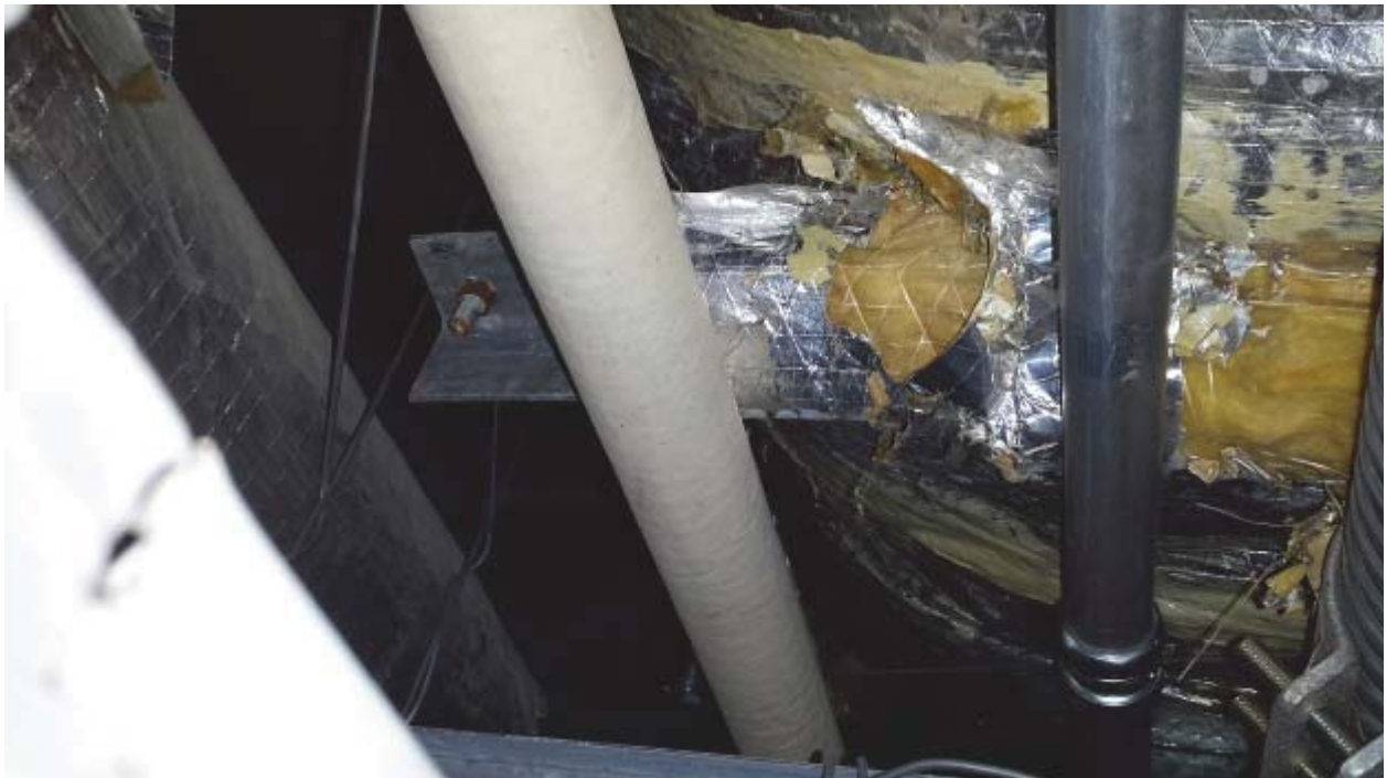
2. Brown/Beige Duct Sealant on Foil Wrapped Duct Insulation with Fiberglass (HM #2)
