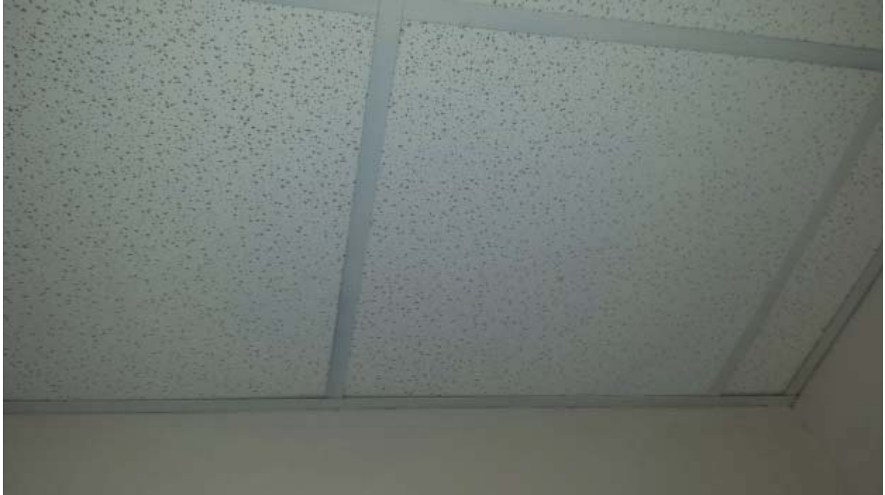
1. White 2' X 2' Ceiling Tile, Small Gouges and Pinholes (HM #1)
