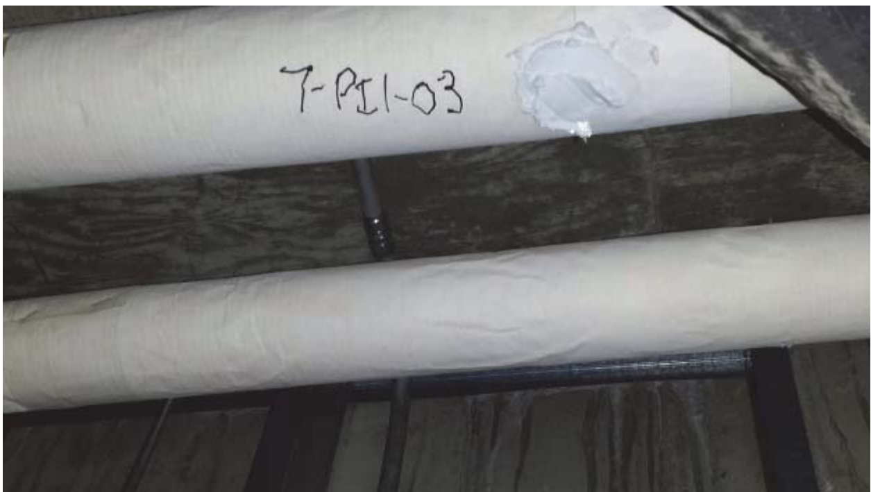
4. Paper Wrapped Pipe Insulation, Fiberglass Confirmation (HM #4)
