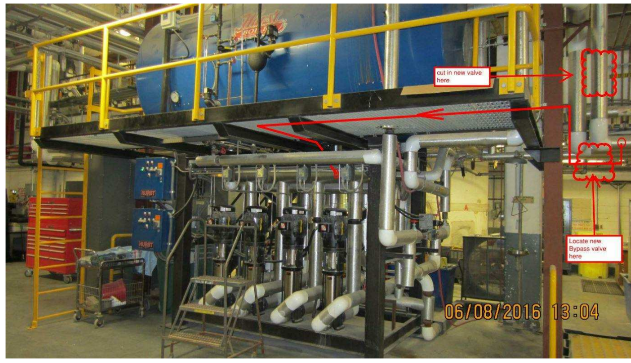
1 DEAERATOR CONDENSATE BYPASS NOT TO SCALE
