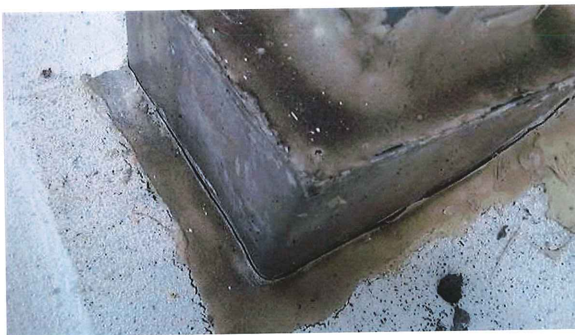
PP-152 Pitch Pan- Sealant failure
