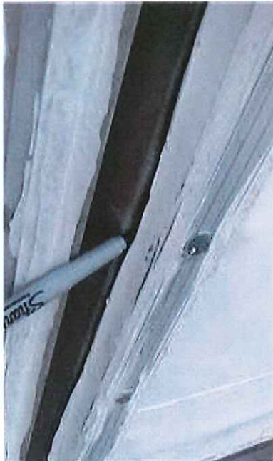
BF-152 Base Flashing- sealant failure
