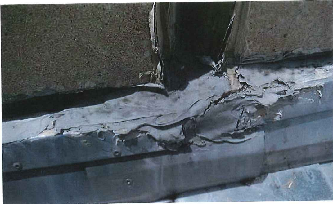
CF-310 Counterflashing- sealant failure
