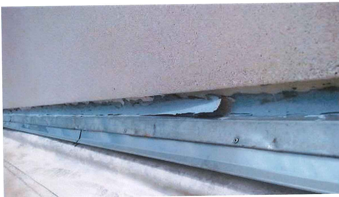
CF-310 Counterflashing- sealant failure
