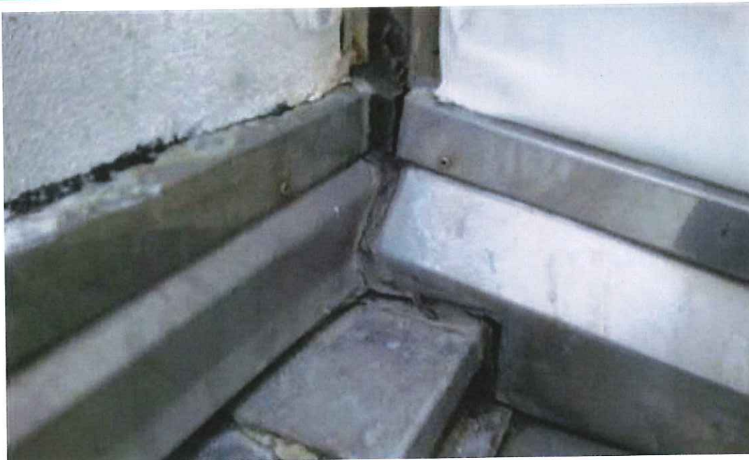
MC-310 Metal Cap- sealant failure
