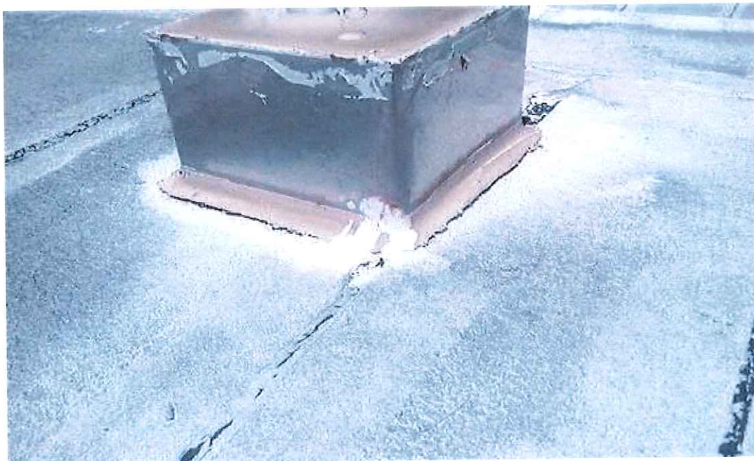
PP-152 Pitch Pan- Sealant failure
