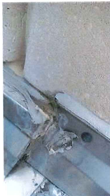
CF-310 Counterflashing- sealant failure
