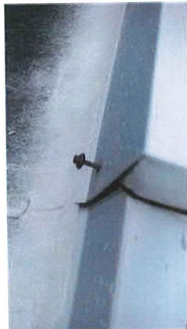
MC-300 Metal Cap- loose/missing fasteners
