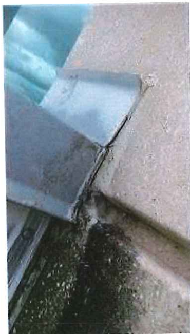
MC-310 Metal Cap- sealant failure
