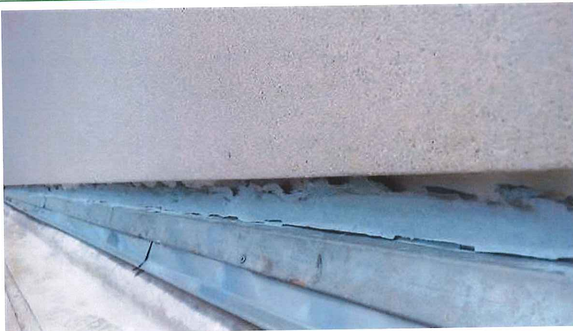
CF-310 Counterflashing- sealant failure
