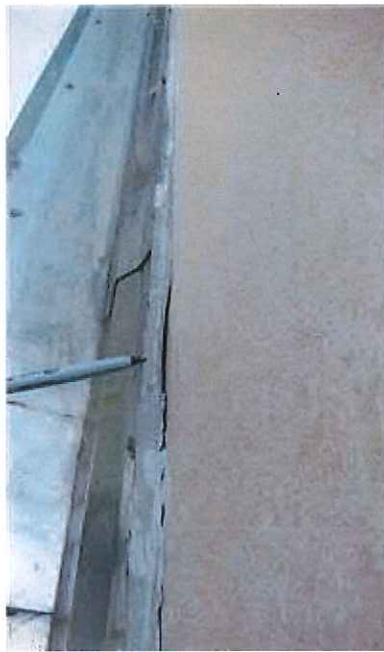
CF-310 Counterflashing- sealant failure
