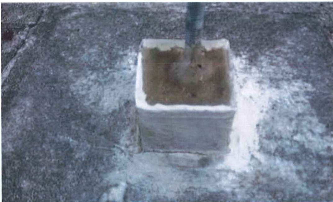
PP-200 Pitch Pan- sealant inadequate
