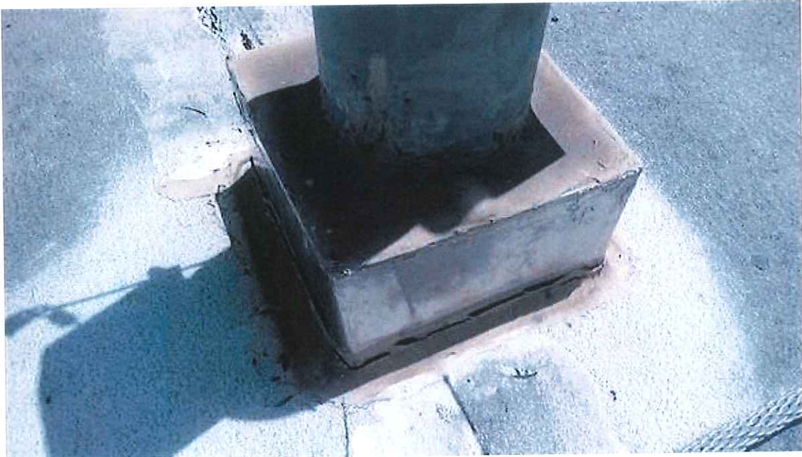
PP-152 Pitch Pan- Sealant failure
