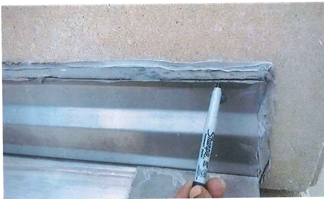
CF-310 Counterflashing- sealant failure
