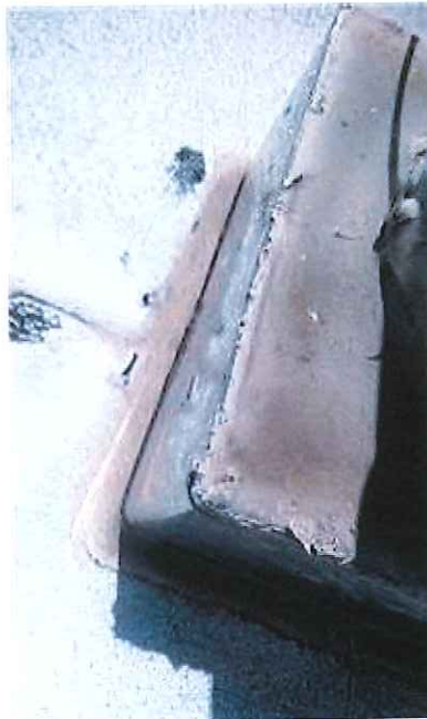
PP-152 Pitch Pan- Sealant failure
