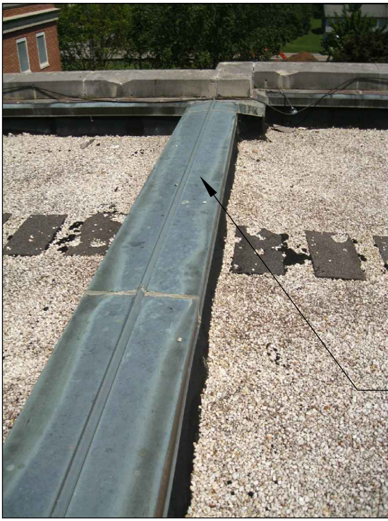
EXISTING EXPANSION JOINT ON ROOF
