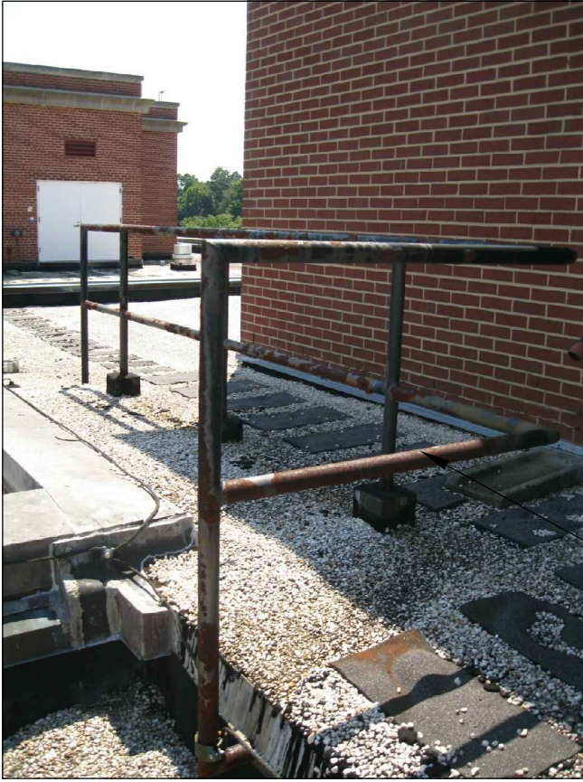
REMOVE AND SAND ALL EXISTING HANDRAILS AND REPAINT.
