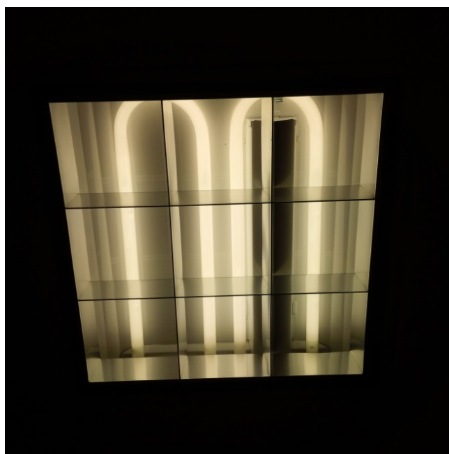
Figure 6 – U-Tube Fixture in the Canteen
