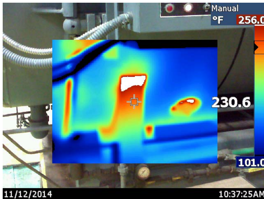
Figure 18 – Uninsulated Boilers
