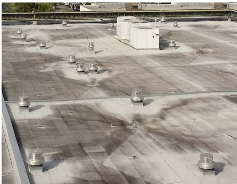
Figure 19 – Exhaust Fans on Roof of M-Deck
