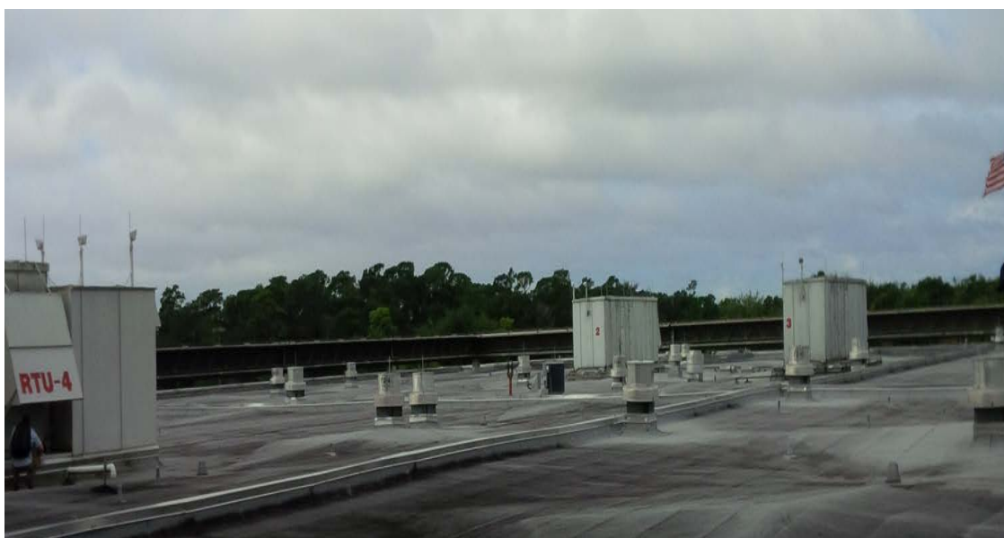
Figure 20 – AHUs on Roof of M-Deck
