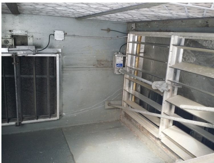
Figure 16 – Improper Economizer Damper Positions
