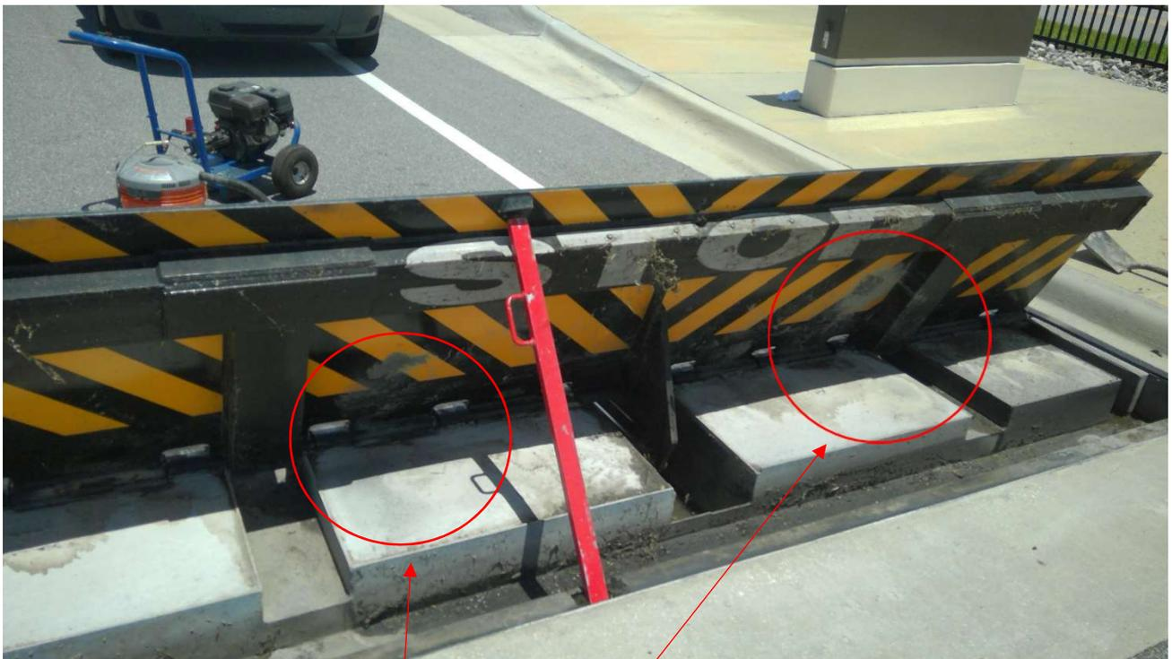
Concrete was poured too high during installation resulting in the plate not resting properly in the down position and also damaging the paint and the galvanizing coating
