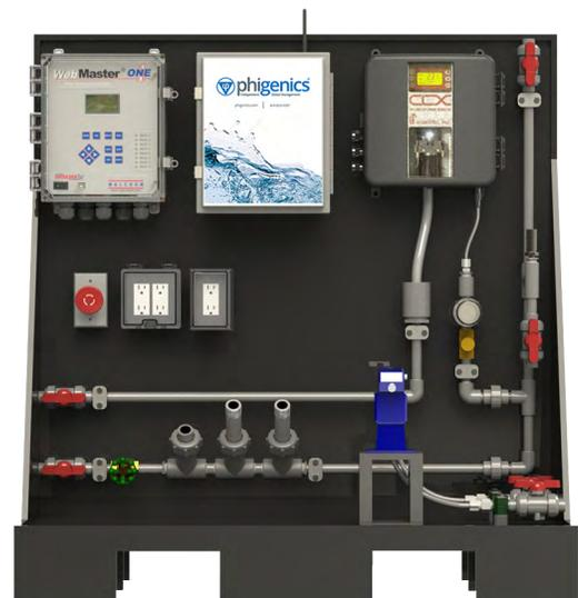
Base Monitor + pH, Temperature, Pressure, Conductivity and ORP-based feed/control of disinfectant
