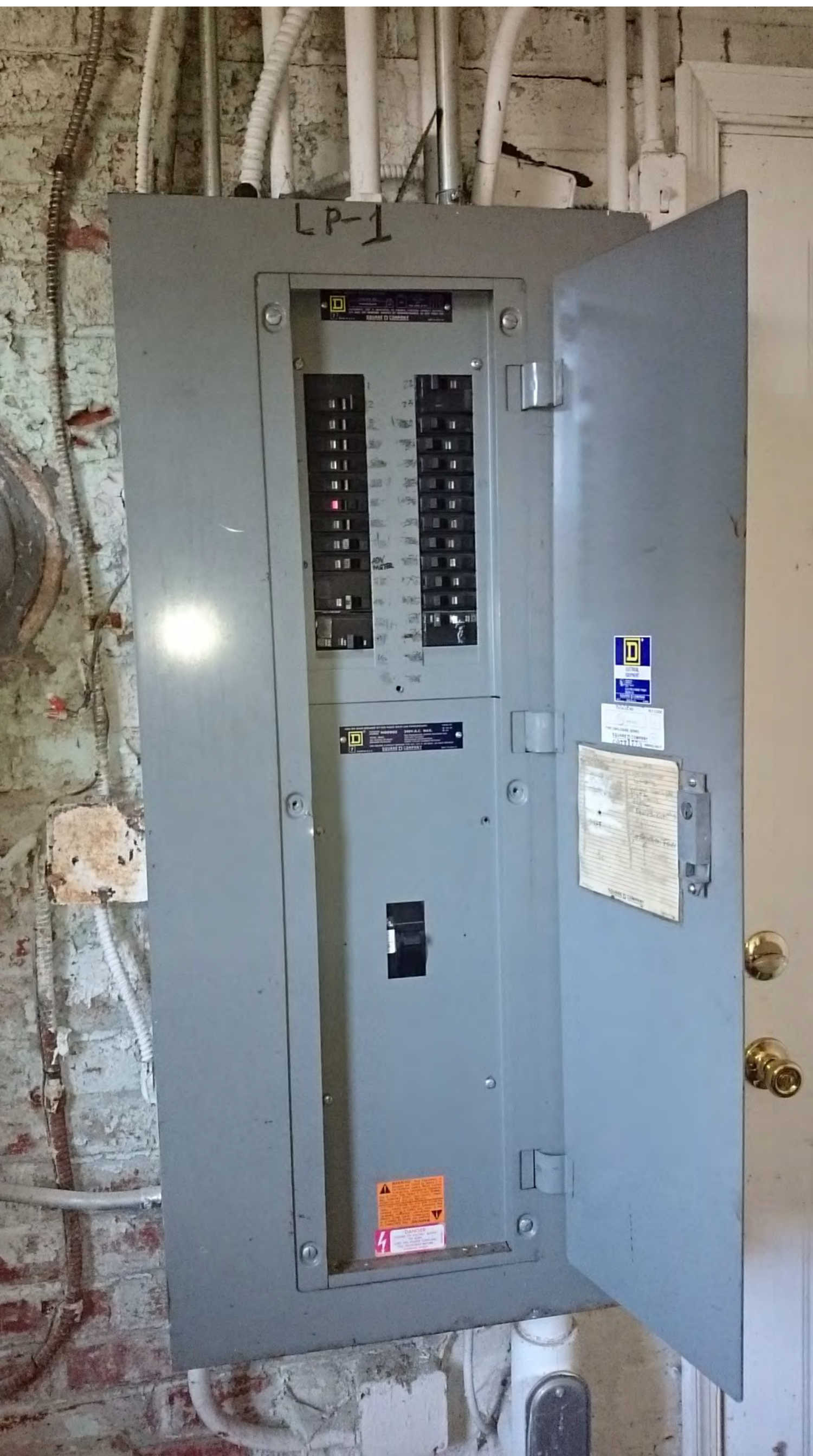
Detail 7: Existing electrical panel. Panel is to be reused, but all existing circuits are to be demolished and replaced with new cable in conduit. See statement of work for more information.
