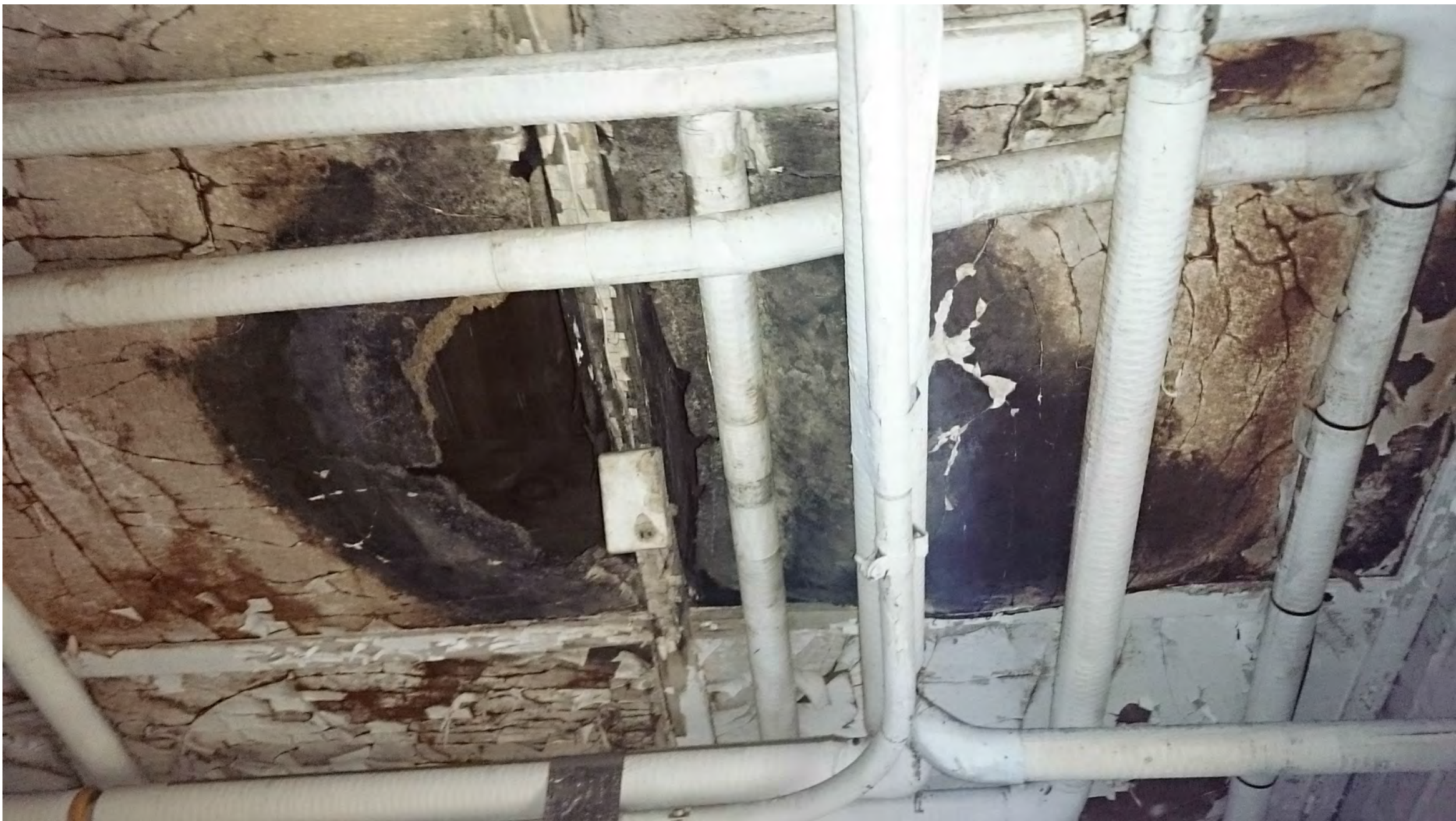
Detail 5: Note area of severe water damage and mold. Demolish ceiling. New work shall not install a new ceiling, but leave an open ceiling plan. Demolish all plumbing, heating, electrical and install new per design build drawing submitted. See specifications for more information.
