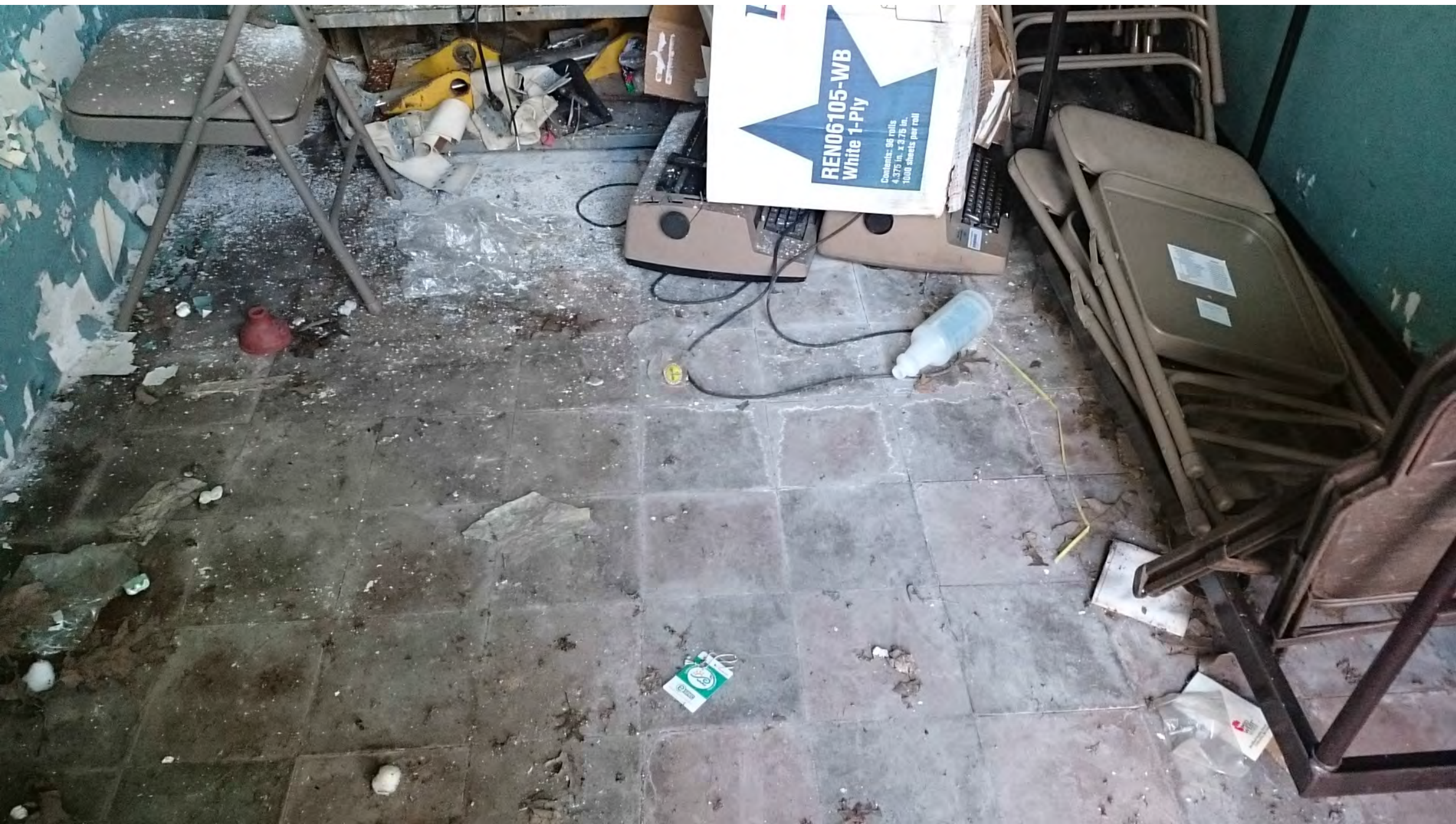
Detail 1: Abate floor, install new VCT. Remove materials, equipment, and trash. Abate lead painted walls, remove drywall, install new drywall and paint.
