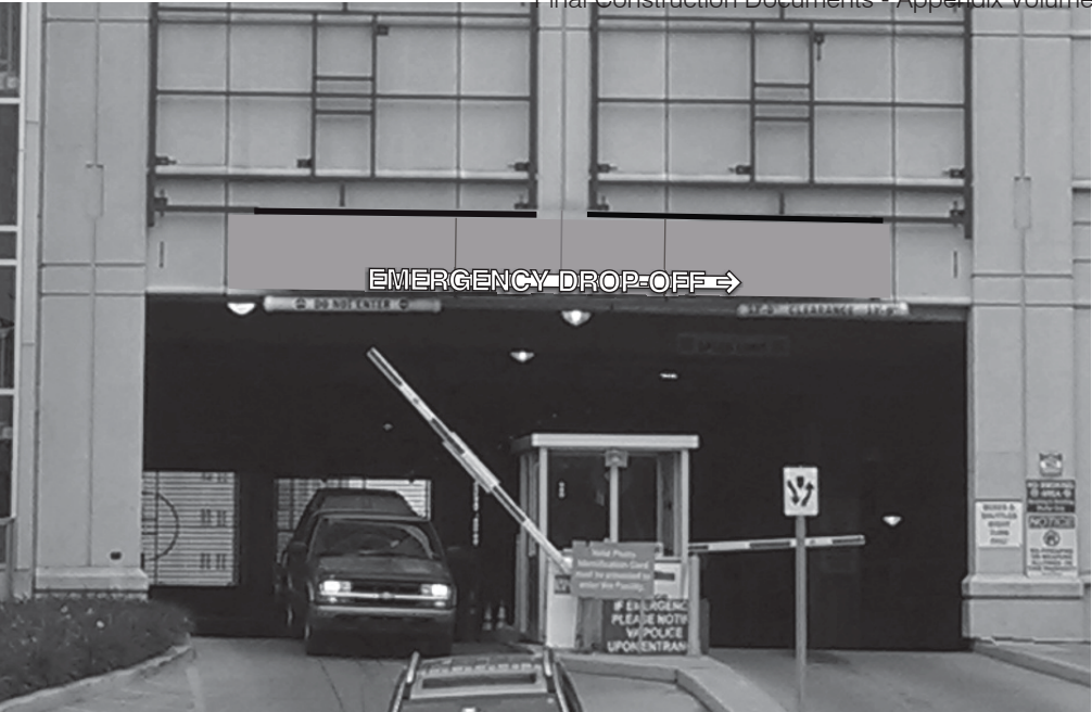
INSTALLATION MOCK-UP Center sign horizontally with vehicle portal Position directly above bullnose of entry portal
