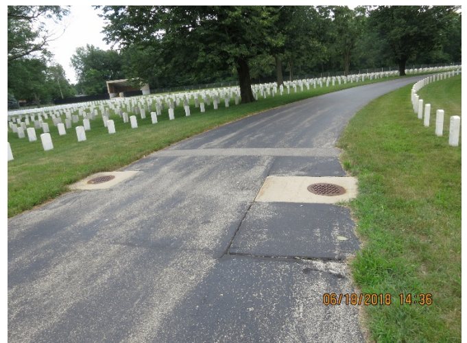
Example of Rim w/Collar in Pavement Area
