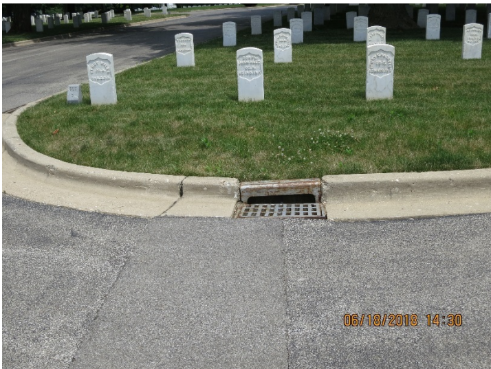
Rim to be Repaired/Replaced
