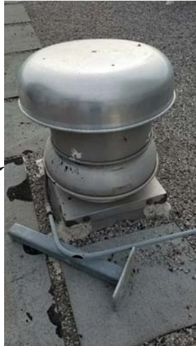
EXISTING ROOF EXHAUST FAN TO BE REPLACED
