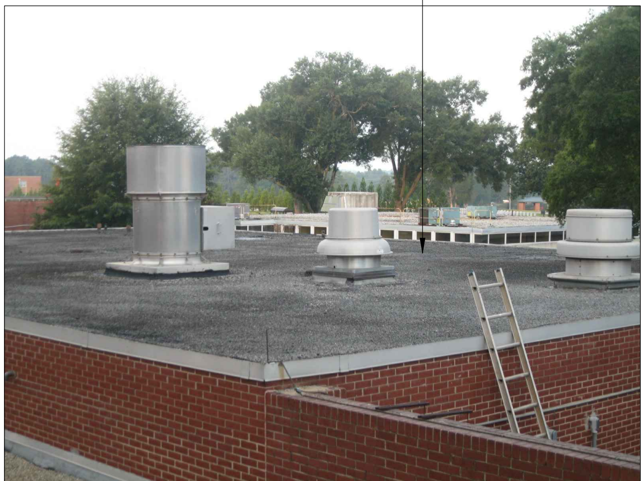
EXISTING BUILDING 31 CHILLER PLANT REMOVE AND REPLACE CURB OR INSTALL NEW CURBS FOR EXHAUST FANS. TYPICAL FOR ALL THREE SECTIONS OF ROOFING OF THE CHILLER PLANT.
