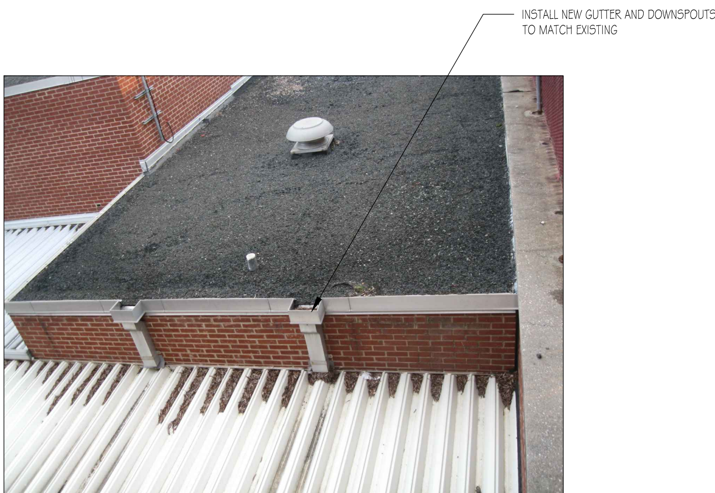
INSTALL NEW GUTTER AND DOWNSPOUTS TO MATCH EXISTING
