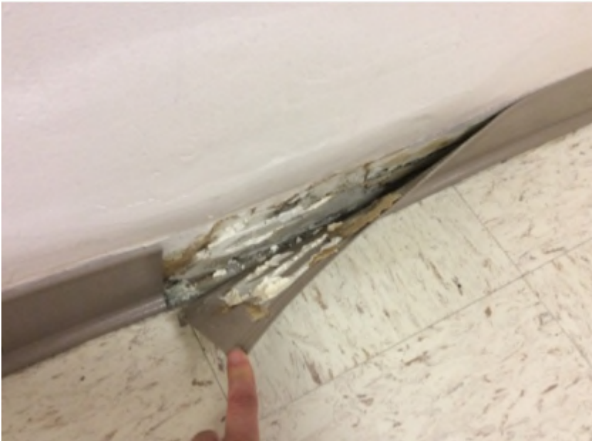
2 nd Floor Corridor Outside Room 2099 – visible moisture damage and suspect staining.
