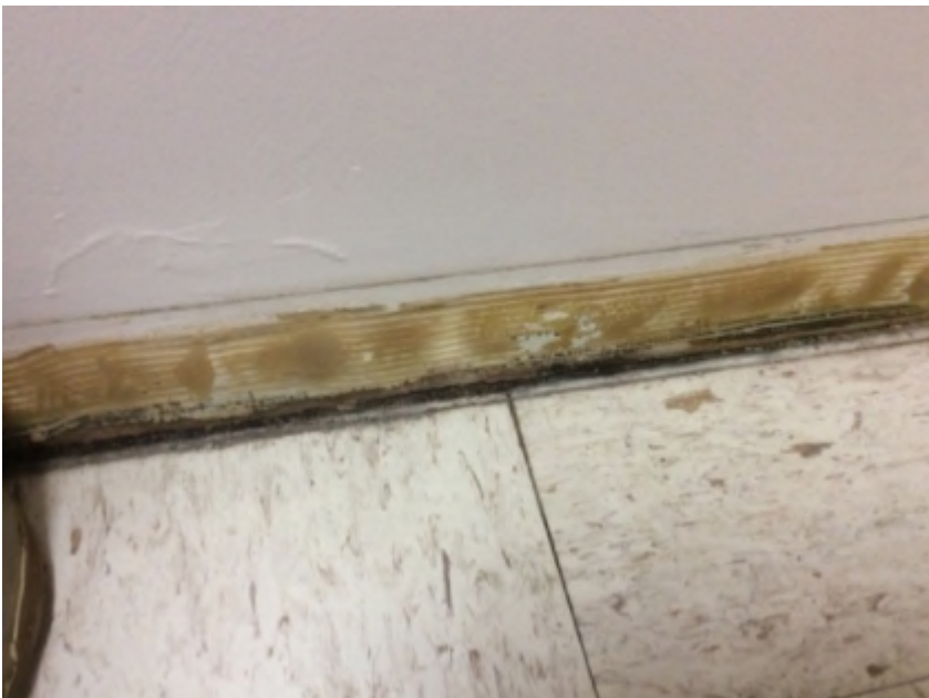
Room 2126 – visible suspect staining on the south wall.
