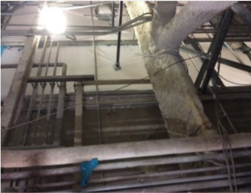
Visible fireproofing debris and stained fireproofing in the interstitial space).
