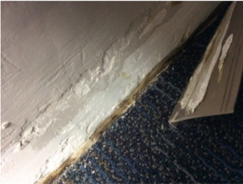
Room 2034 – suspect staining on the south and east wall.
