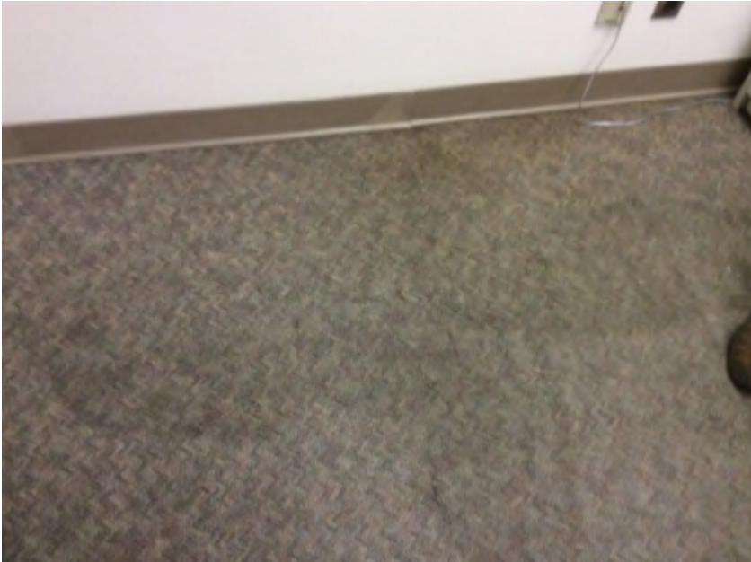
Room 2125 – visible moisture damage on the carpet.
