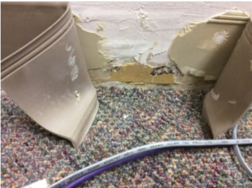
Room 2069A – suspect staining on the east and west wall.
