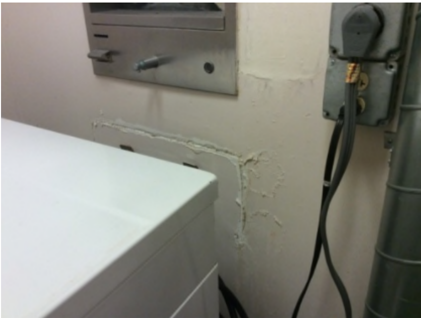
Room 2103 – appears there has been historical moisture damage on the east wall from the washing machine and does not appear to be from the flood incident.
