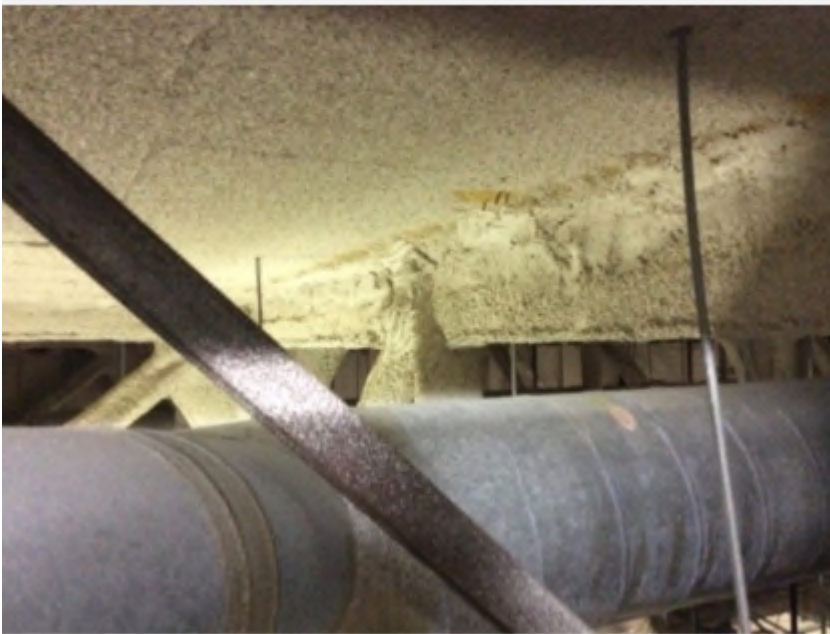
Visible stained fireproofing above Room 2085 and Room 2086.
