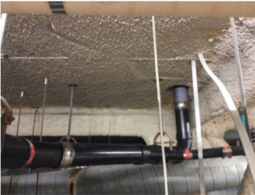
Visible stained fireproofing above Room 2024.
