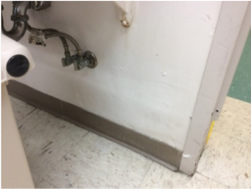
Room 2071 – Appears there has been historical moisture damage on the north wall from the sink and not the flood incident.
