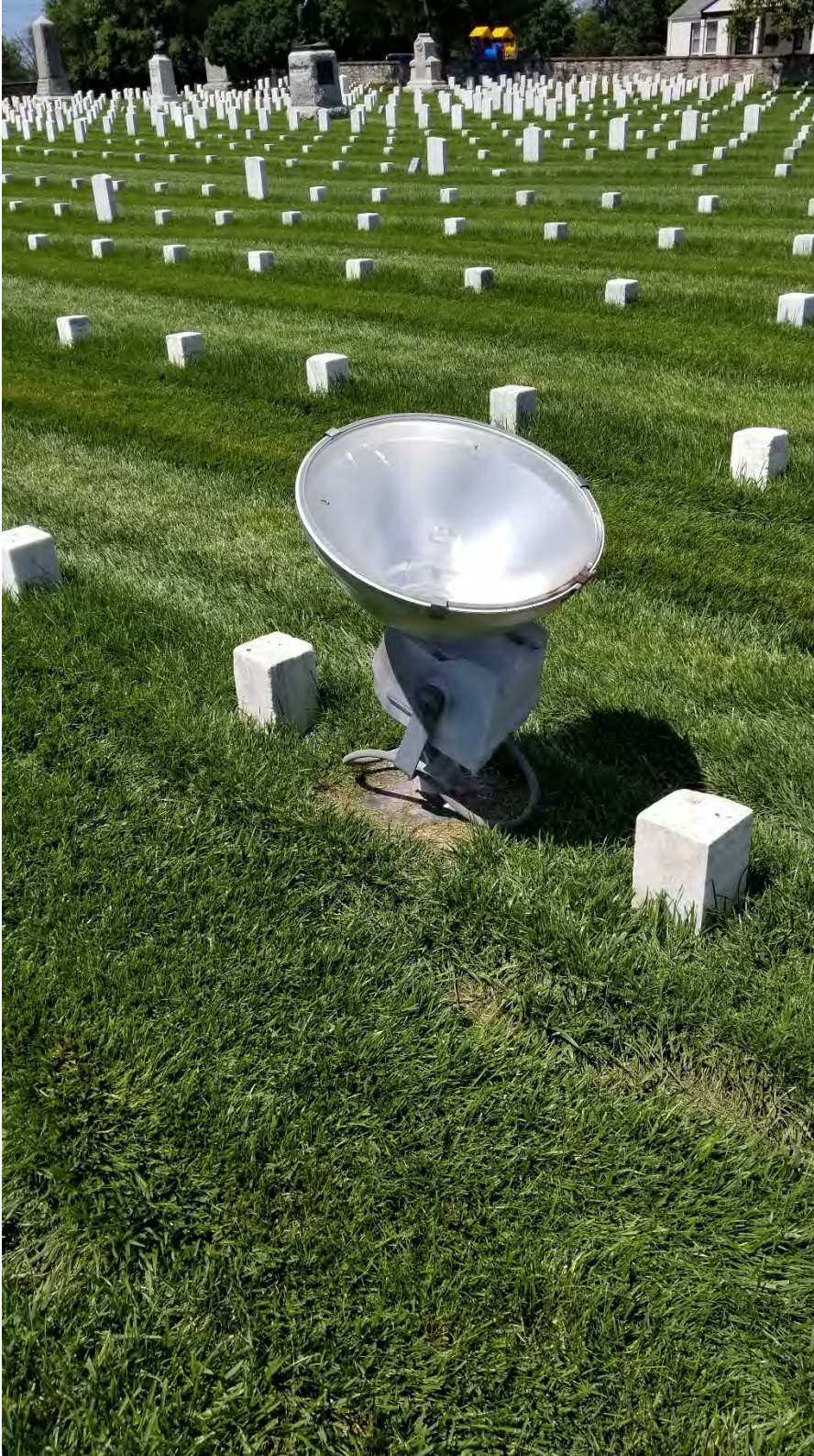
Figure 7: Existing Flagpole Floodlight (typical 3 locations). Note close proximity to existing burial markers. Contractor shall take precautions to protect existing burial markers.
