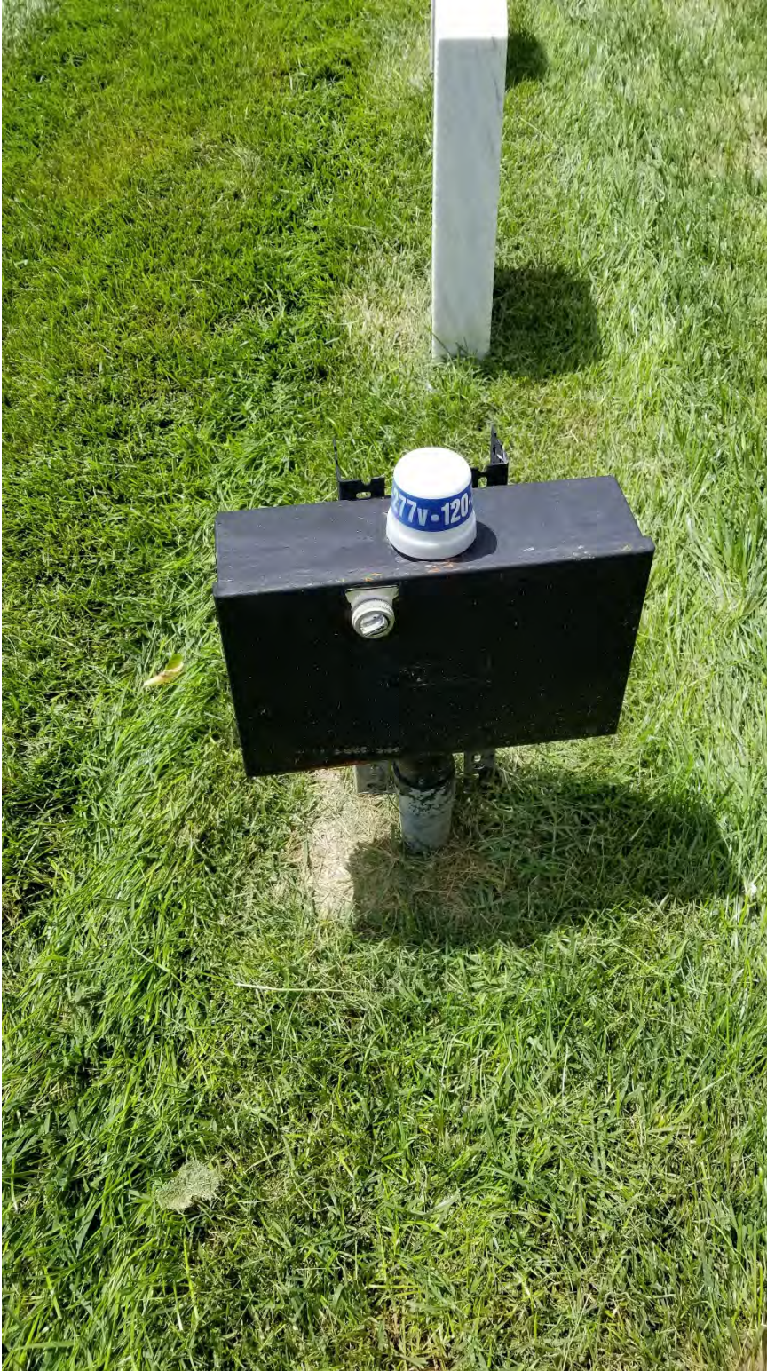
Figure 8: Demolish existing photocell and bypass circuit in this location inside of a new pull box per electrical code. Again, precautions required by contractor to protect existing nearby burial markers.
