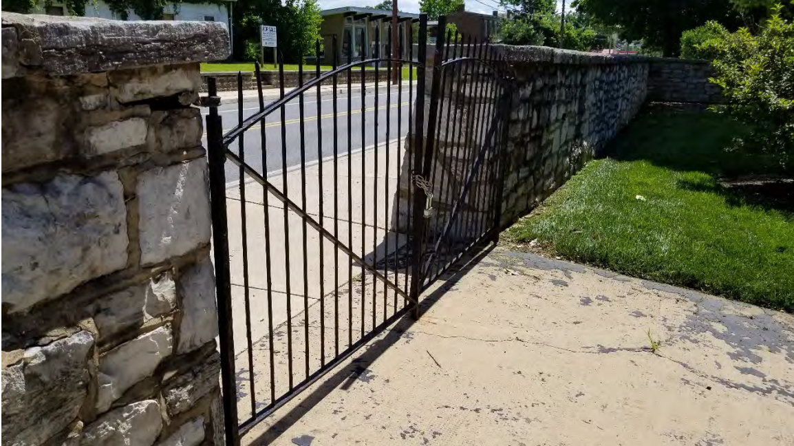
Figure 4: Maintenance Building Gate. Note this gate requires removal, replacement of hardware, and reinstallation to provide a straight and true gate.
