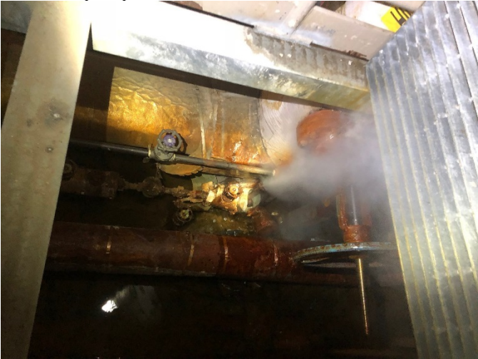
CAPTION 1: BLDG 40 - Crawlspace 3/4-in Drip trap for main line
