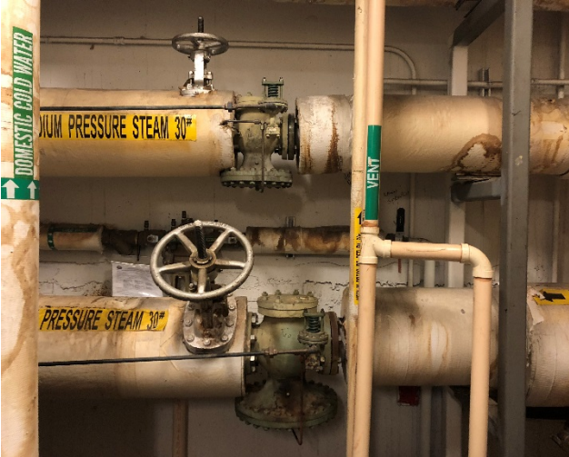
CAPTION 2: BLDG 40 - 1600 3-in (top) 5-in (bottom) Pressure Regulators
