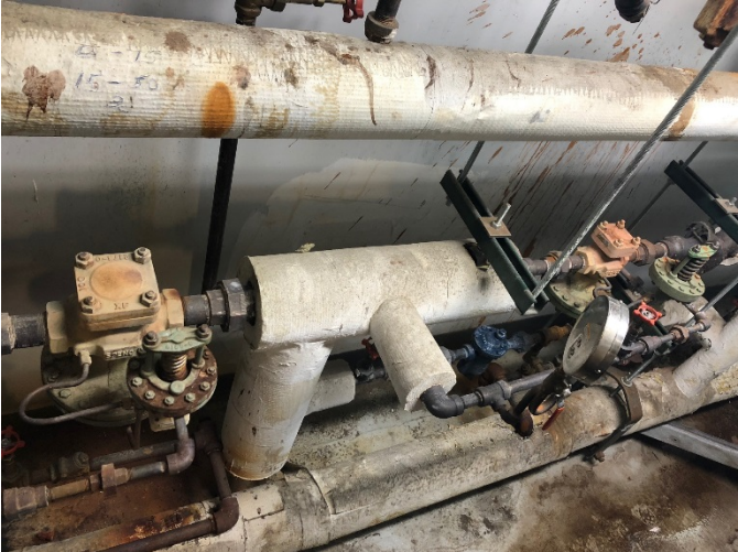
1 1/2-in Pressure regulator (left) 1-in Pressure Regulator (right)
