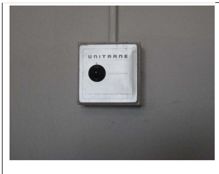
Photograph 12. Air controller – Level 9 – HBM: Potential Mercury.
