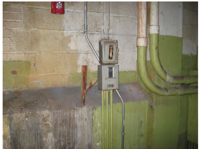
Photograph 8. Electrical Switches– Penthouse mechanical room – HBM: Potential Mercury.
