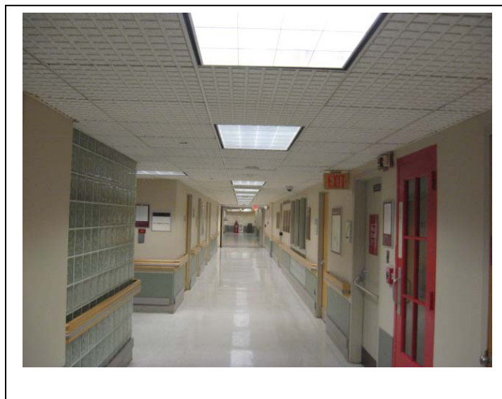
Photograph 16. Florescent bulbs and ballasts – Level 1 – HBM: Mercury and PCBs.
