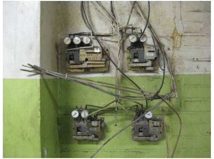
Photograph 6. Pressure gauges– Penthouse mechanical room – HBM: Potential Mercury.
