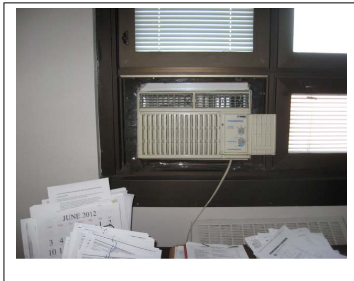
Photograph 14. Air-conditioner – Level 9 – HBM: CFCs related to refrigerant.
