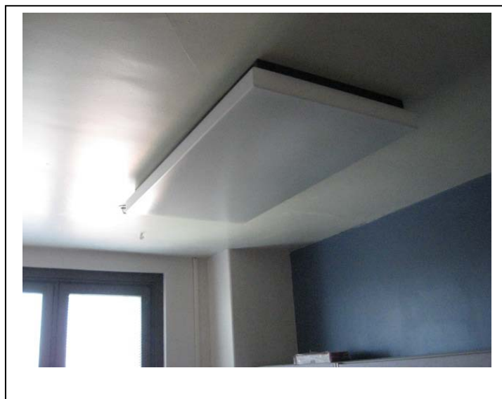
Photograph 11. Florescent bulbs and ballasts – Level 9 – HBM: Potential Mercury and PCB.
