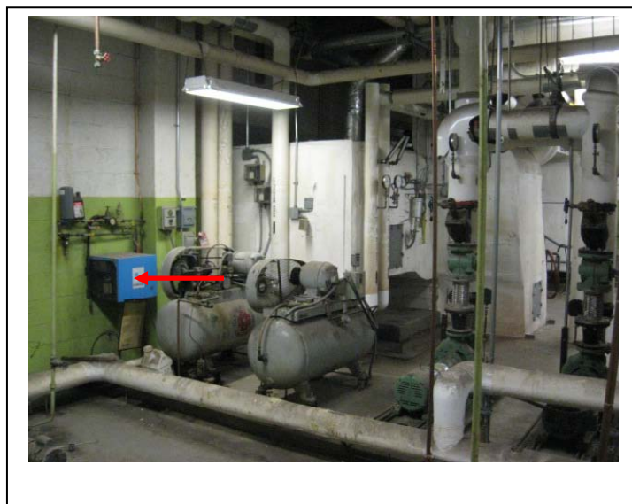
Photograph 9. Compressed air drier – Penthouse mechanical room – HBM: Refrigerant R134A or R22
