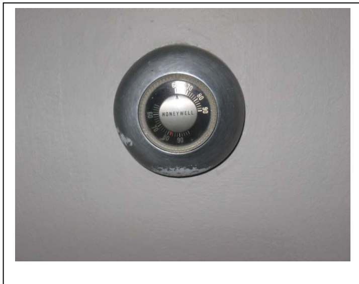
Photograph 13. Thermostat – Level 9 – HBM: Potential Mercury.
