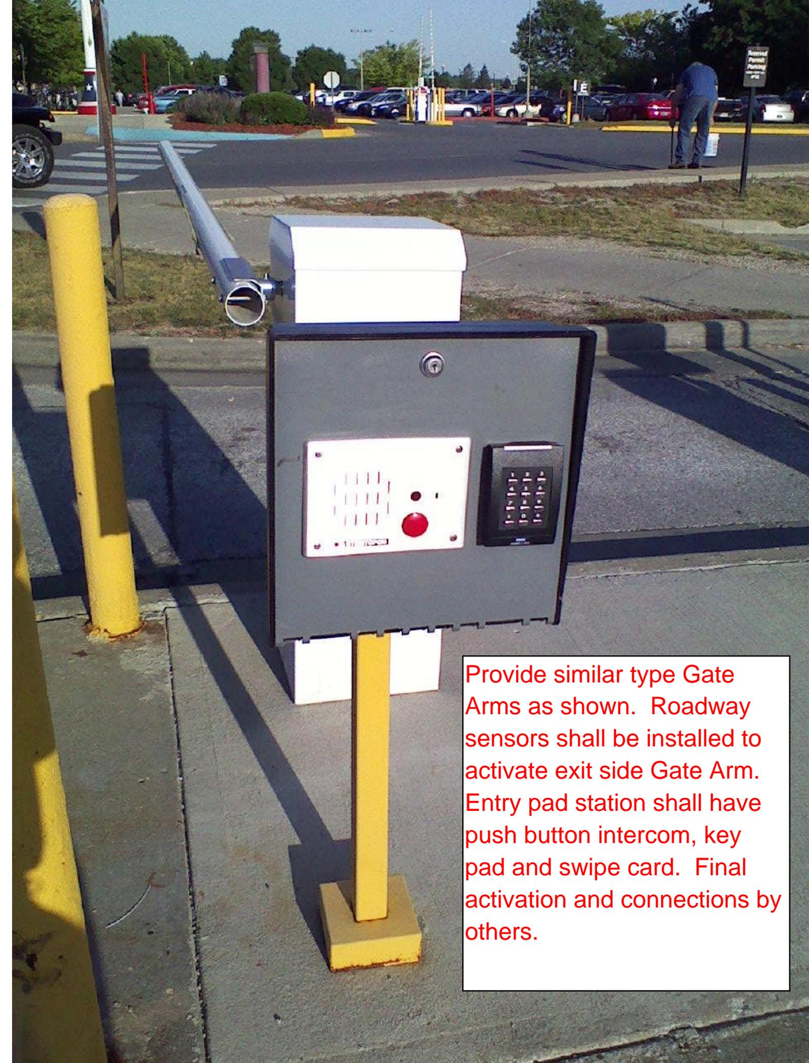
Provide similar type Gate Arms as shown. Roadway sensors shall be installed to activate exit side Gate Arm. Entry pad station shall have push button intercom, key pad and swipe card. Final activation and connections by others.
